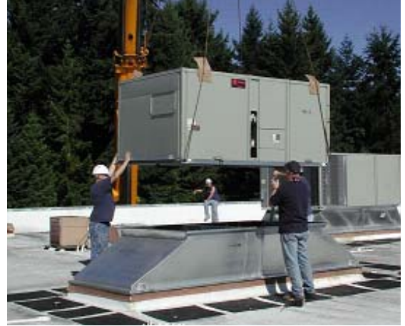
Installing a commercial rooftop HVAC
