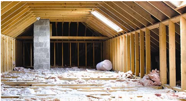
A typical attic insulation project.
