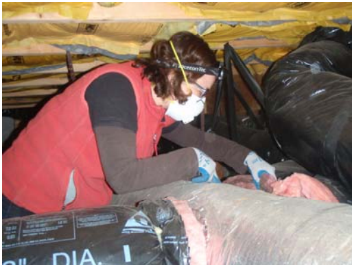
A PSE QA inspector reviews duct insulation.
