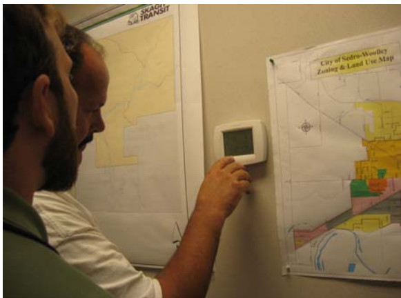
A facility manager checks thermostat settings during RCM walk-through training.
