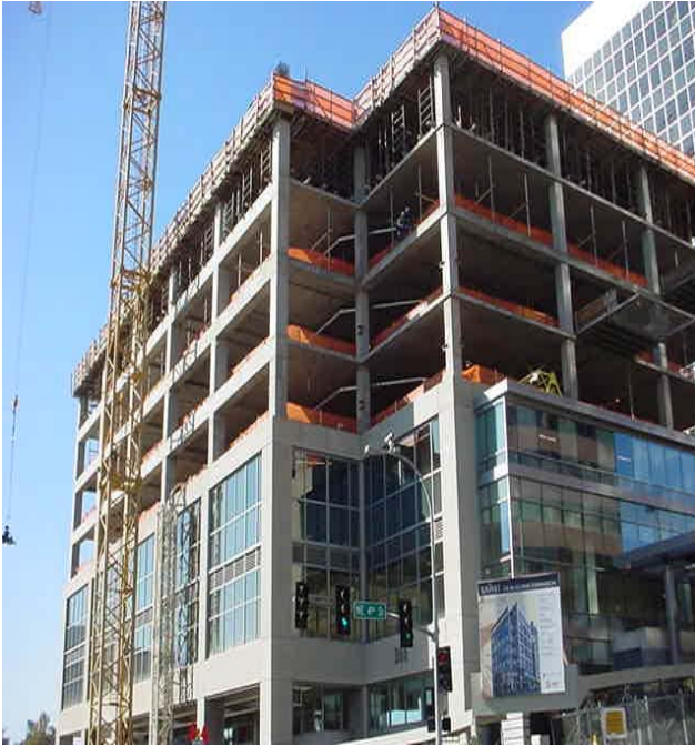
The PSE campus's EST building under construction.
