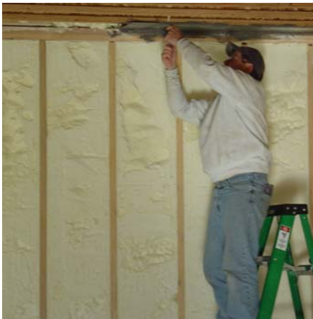
A wall insulation job using sprayed foam.
