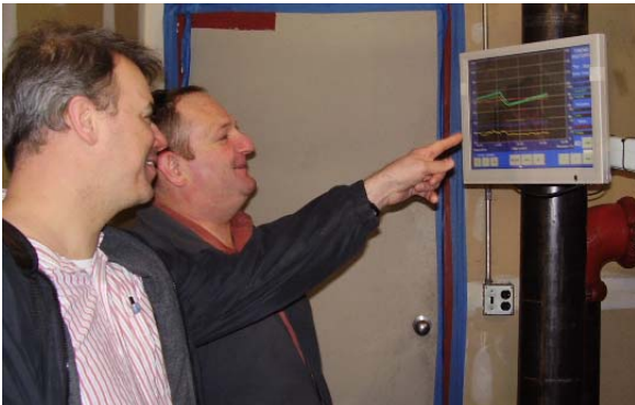
A PSE EME verifies performance of newly installed equipment.
