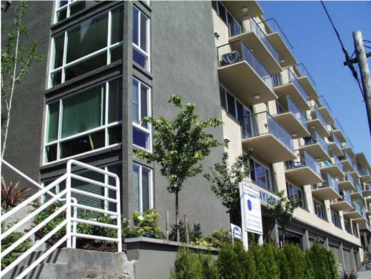
A typical newly-constructed multifamily structure.
