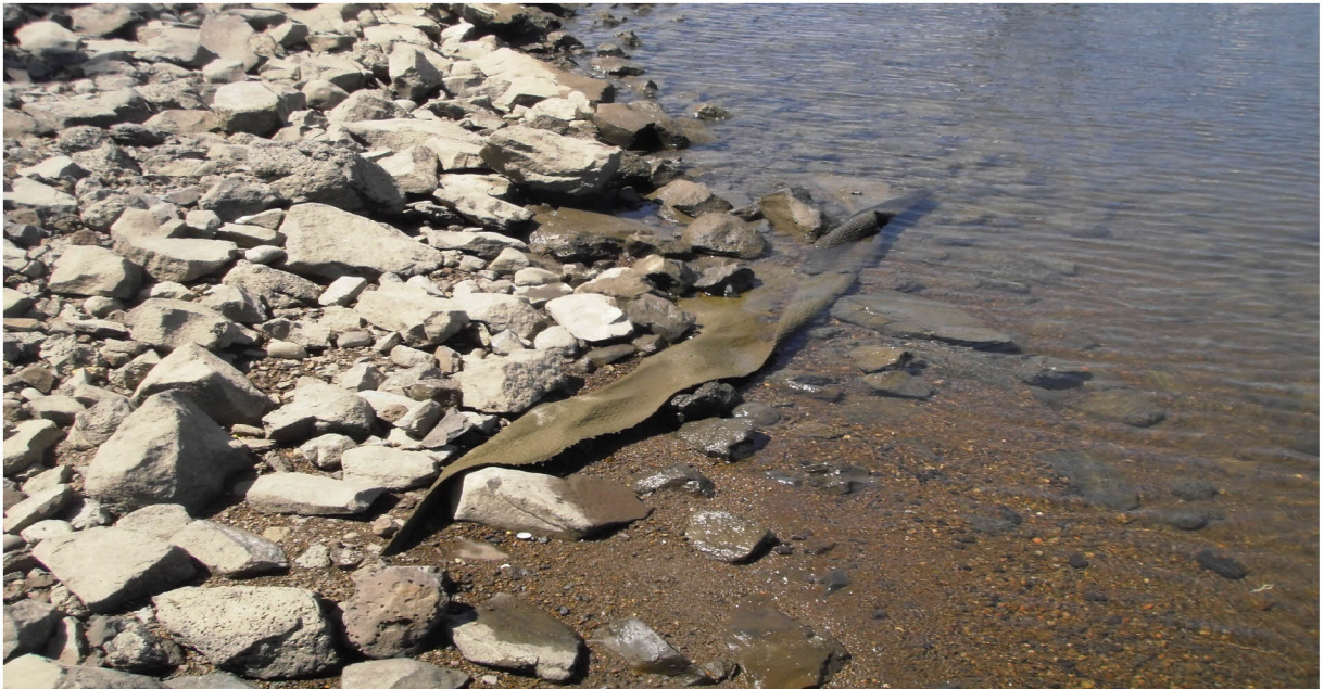
Photo 2 Exposed Organoclay Mat Material at the Shoreward Lateral Midpoint of Cap (7/23/2020)
