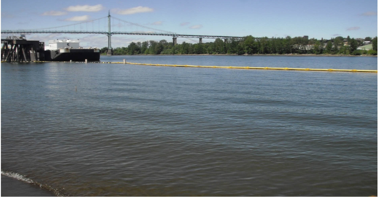
Photo 1 PacTerm Oil Boom Placement from Dock to Dolphin with Three Mariner Warning Buoys at Pilot Cap Area (7/23/2020)
