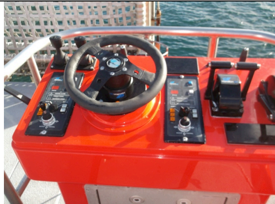
08 Aft Control Station
