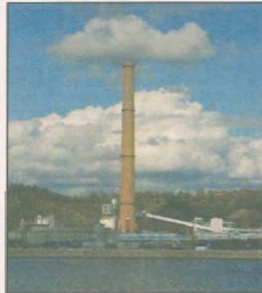
PORT OF TACOMA PHOTO
