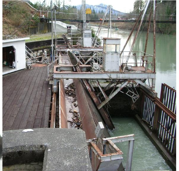
**Old trashrack and intake for Powerhouse 2, needs rebuild and upgrade for new weir elevations**
