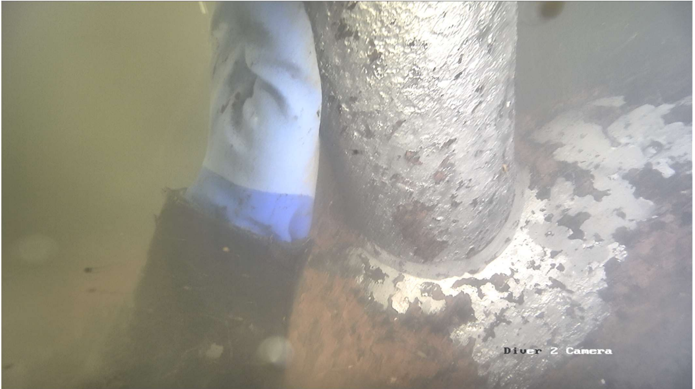
Figure 8 - Weld connection diffuser #1
