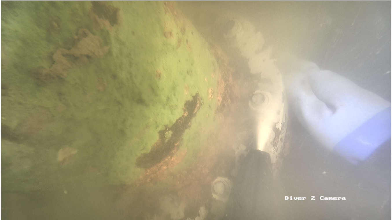
Figure 4 - AAC Diver cleaned the hardware and connections.
