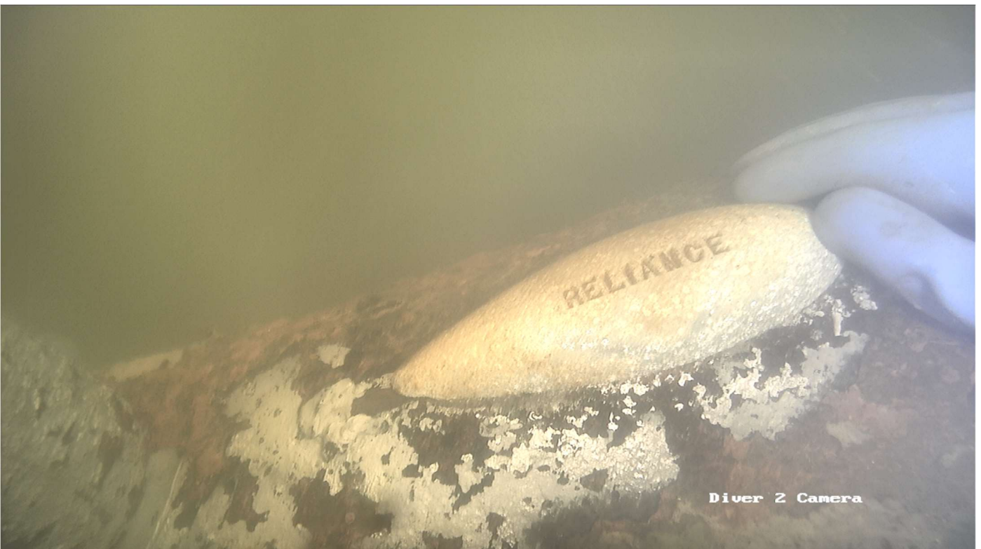
Figure 7 - Sacrificial anode in good condition.
