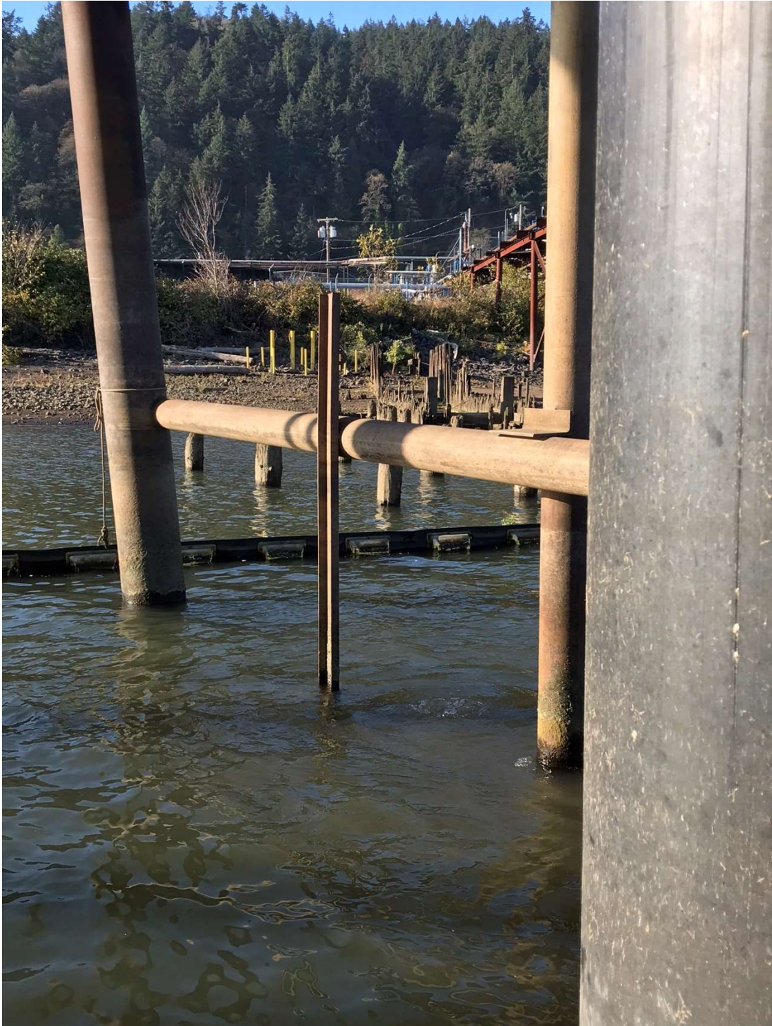
Figure 3 - Outfall channel iron support.
