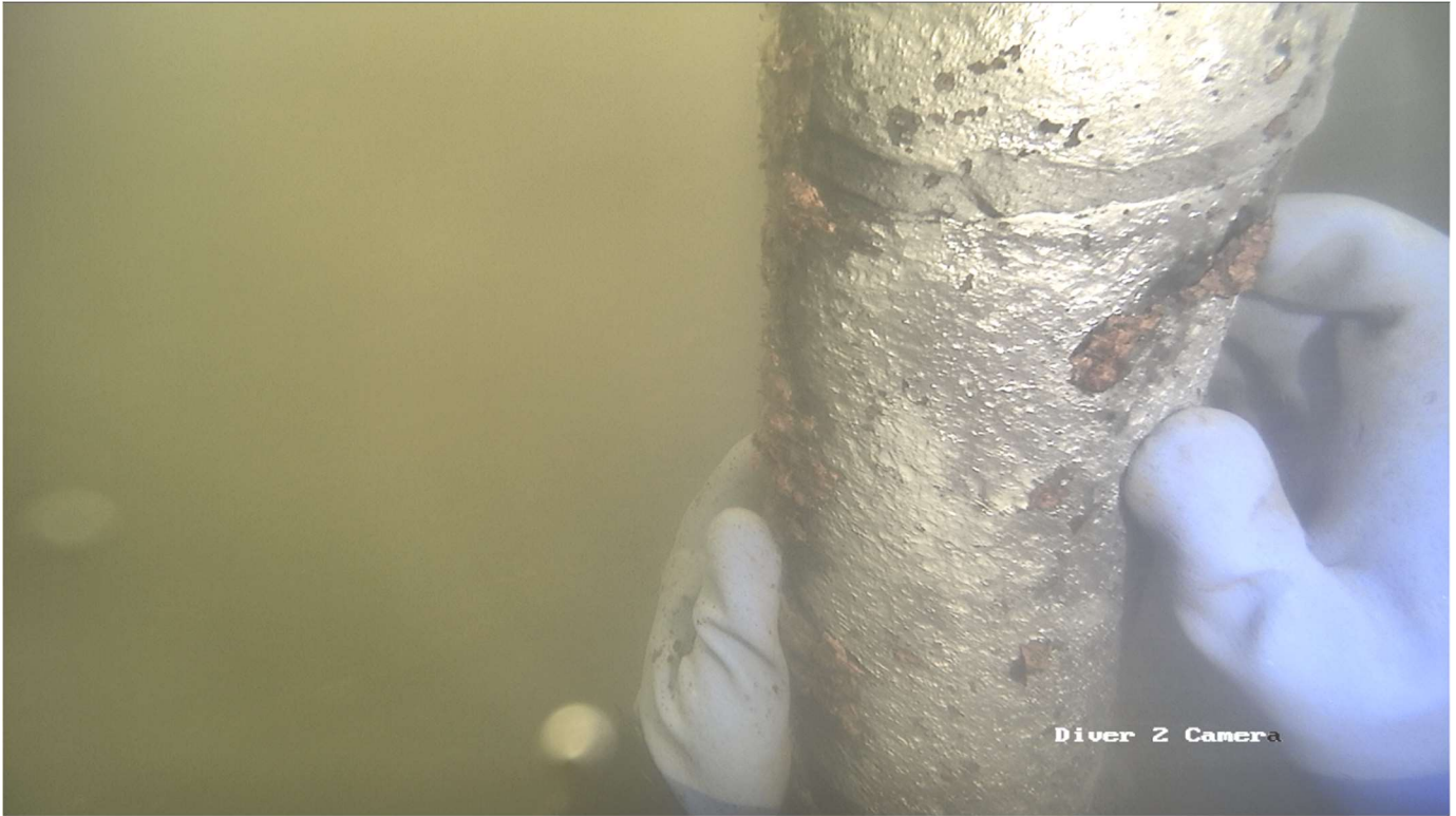
Figure 9 - Minor pitting present (typical).
