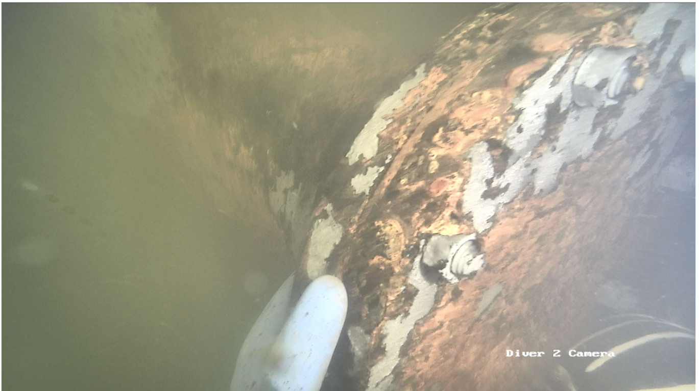
Figure 6 - Blind flange hardware in good condition.
