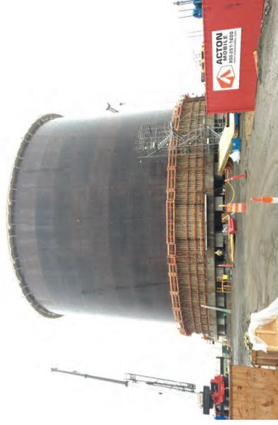
Form work for first concrete tank ring complete
