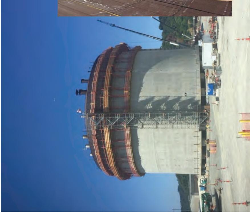
Completed pour of outer tank ring #7 (out of 8)
