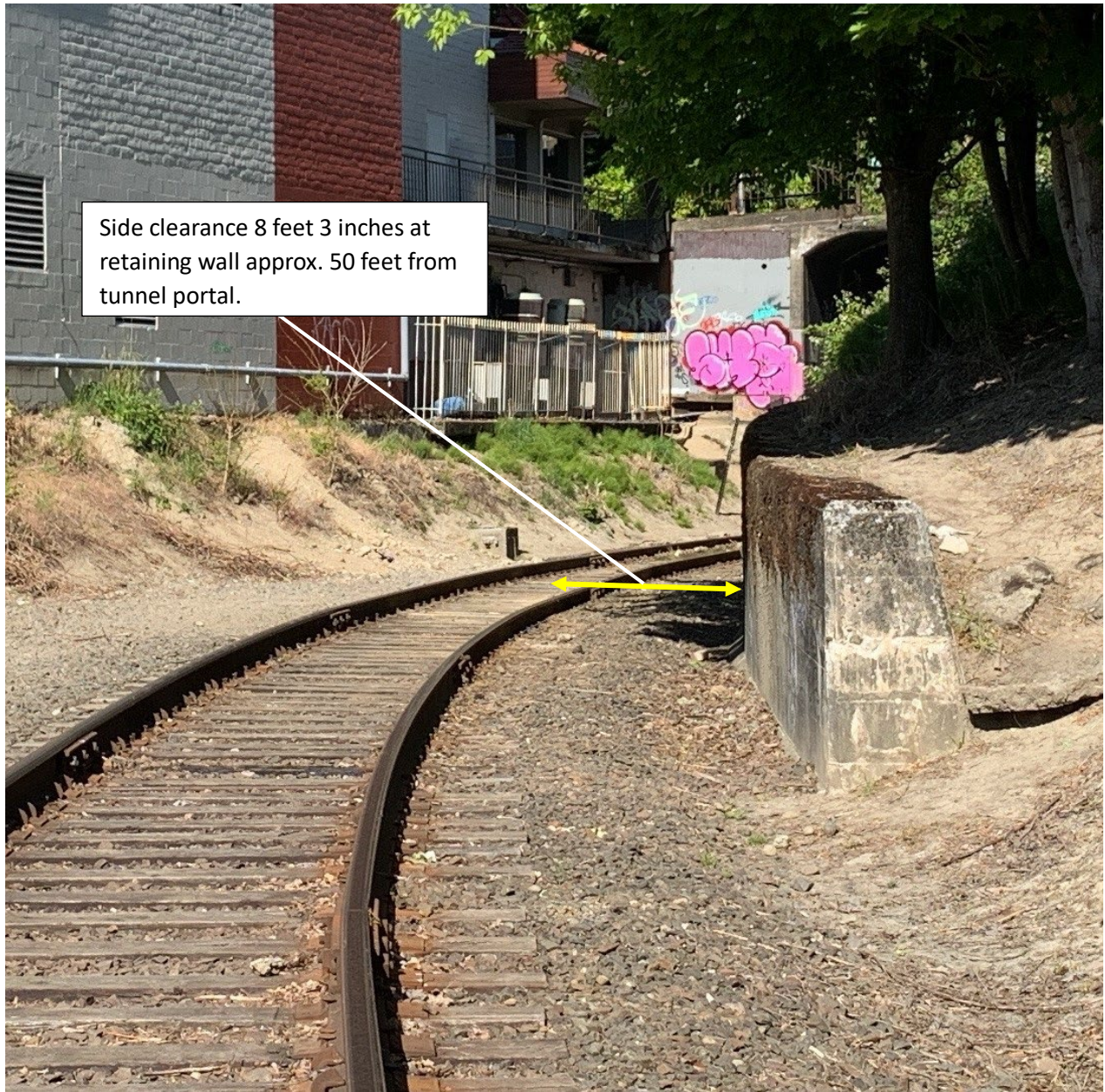
Retaining wall at curve on west approach
