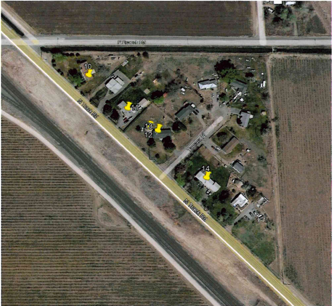
Figure 4: Section of the proposed pipeline showing buildings 10 - 14 within the 100-foot proximity boundary.
