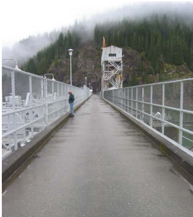
Photo 8 – View to the north along access road across top of Upper Baker Dam
