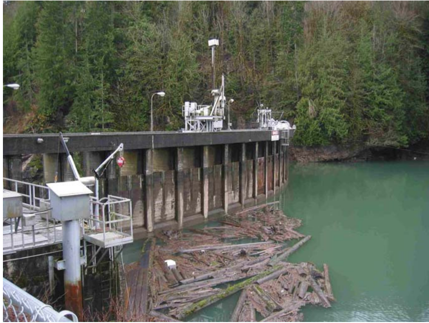
Photo 3 – View looking at upstream face of Lower Baker Dam, showing spillway gates in closed position. Water level is about 3 feet below crest. Reservoir elevation recorder in lower left corner adjacent to penstock intake structure.
