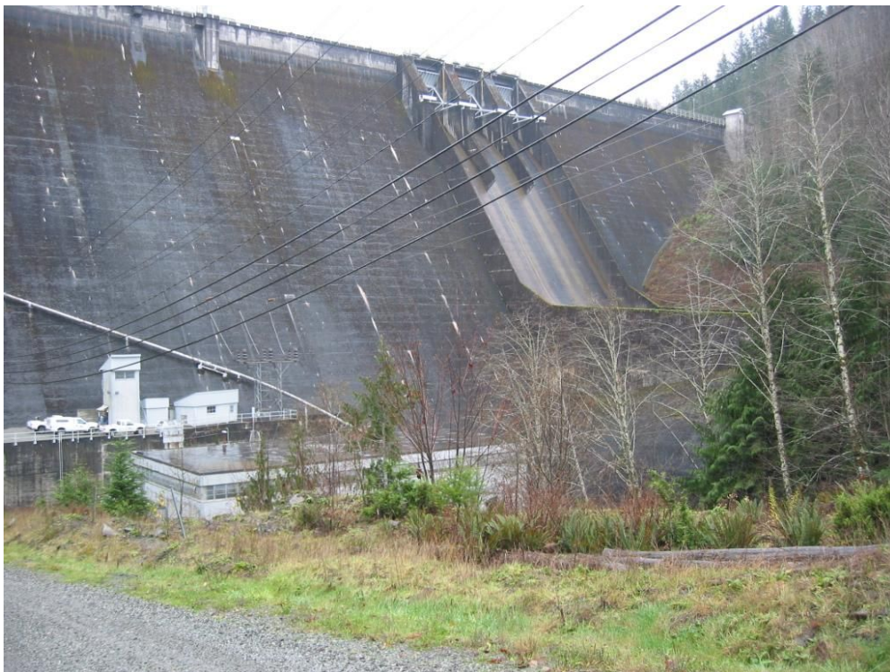
Photo 2 – View of downstream face of Upper Baker Dam (powerhouse in foreground)
