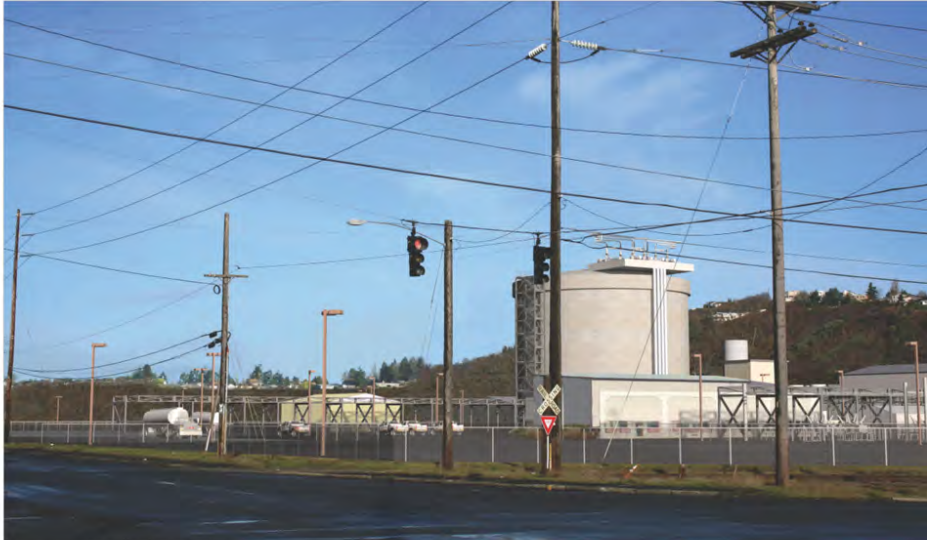
PSE's Tacoma LNG Facility, to be completed by 2018
