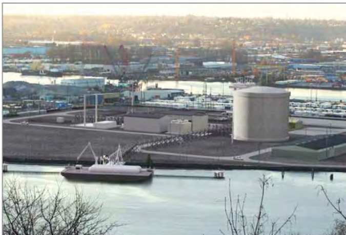
PSE's Tacoma LNG Facility, to be completed by 2018
