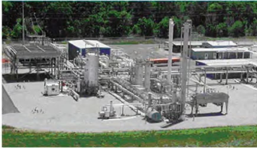
Figure 10: Single Mixed Refrigerant LNG Facility
