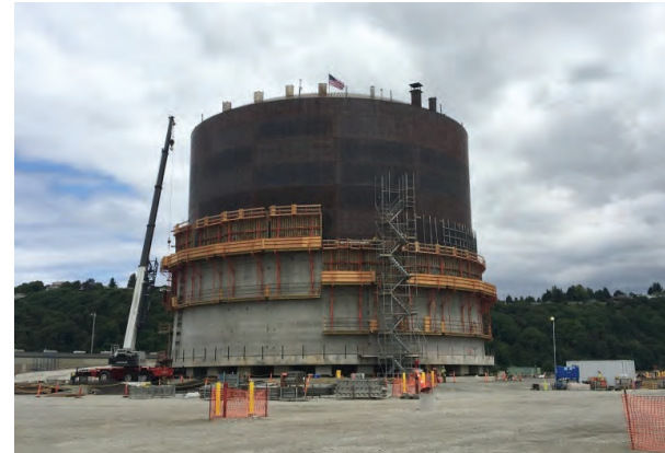
Three of eight concrete tank ring completes
