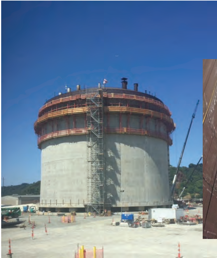
Completed pour of outer tank ring #7 (out of 8)
