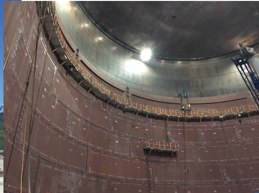
Installation of inner tank ring #8 (out of 10)
