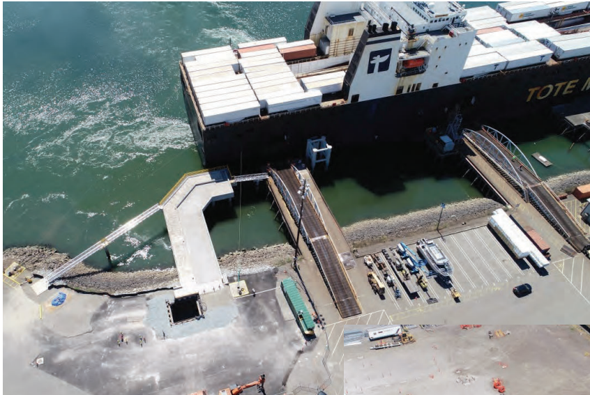
Completed fueling pier
