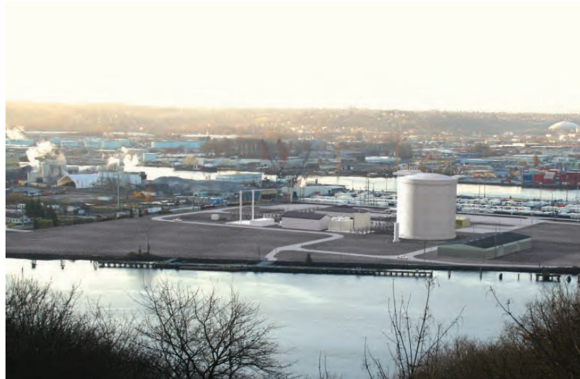
Tacoma LNG facility in Tacoma, Washington
