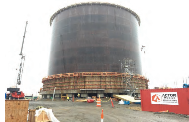
Form work for first concrete tank ring complete
