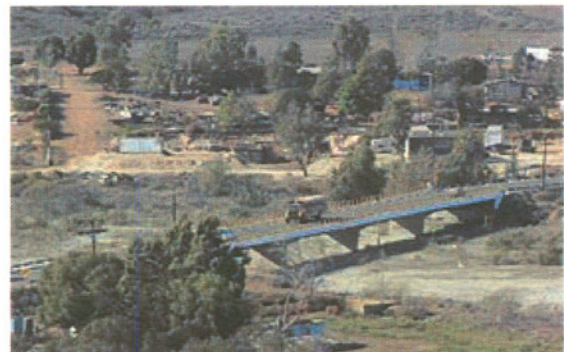
CHARLIE NEUMAN / Union-Tribune In Colonet, a bus crossed over the San Rafael River, which empties into the ocean at Punta Colonet when the river is flowing.
