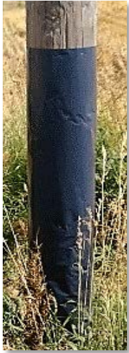
Fire mesh can last more than 20 years and requires no maintenance.
