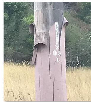
Fire resistant paint tends to fail in about 3-5 years and must be reapplied.
