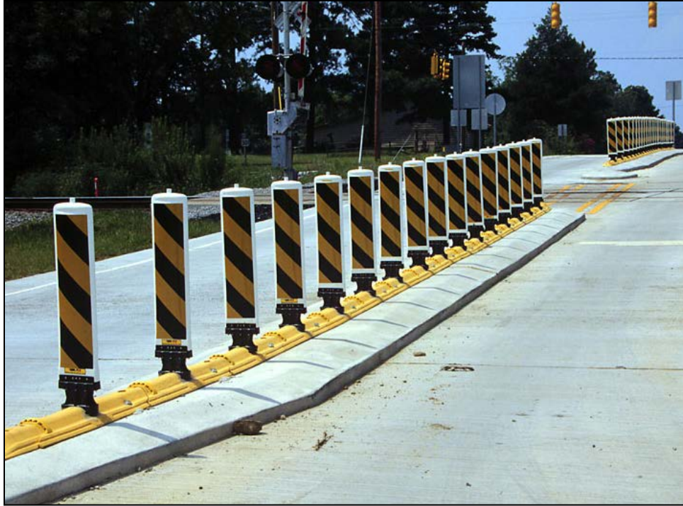
Figure 3. Mountable Raised Curb System with Vertical Panels ( photo courtesy of NCDOT )
