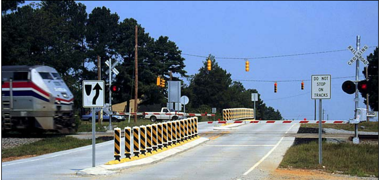
Figure 1. Traffic Channelization Device Installation at Highway-Rail Grade Crossing (photo courtesy of NCDOT)
