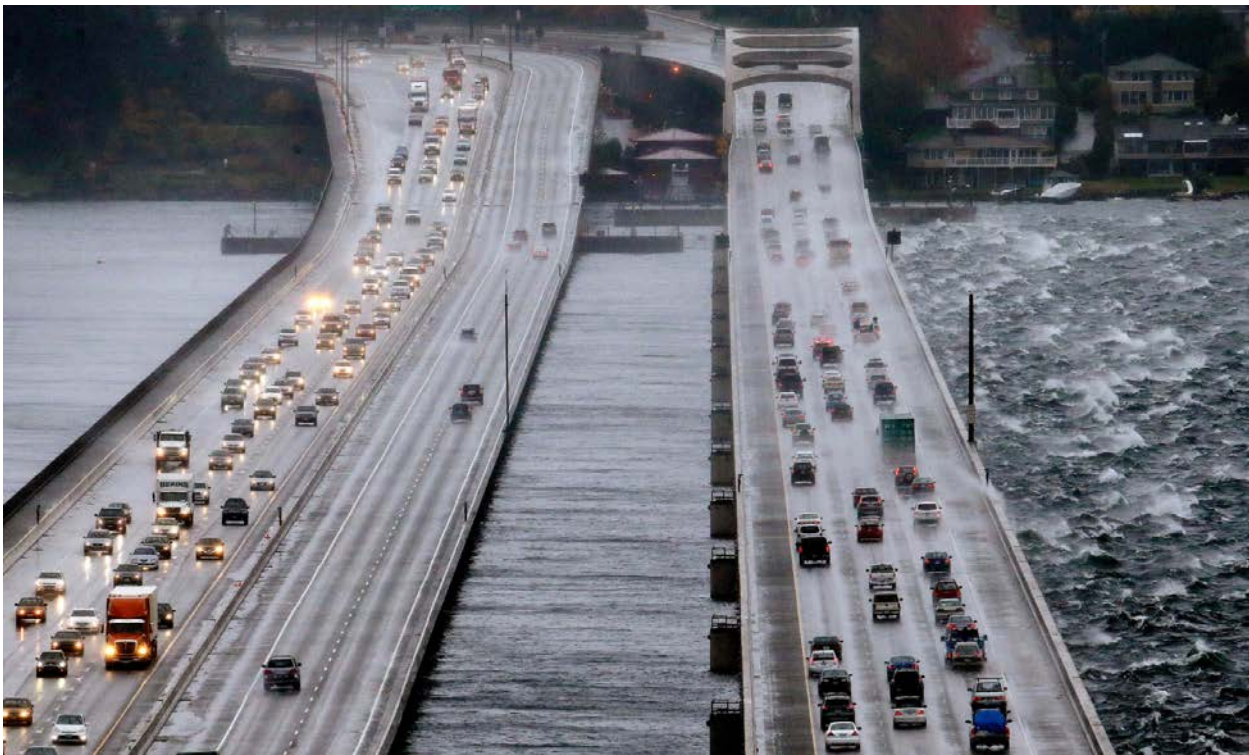
Eastbound traffic lanes, right, on Interstate 90 are dampened by wind-driven waves from the south as the floating bridge calms Lake Washington to the north on Tuesday. Photograph: Elaine Thompson/AP
