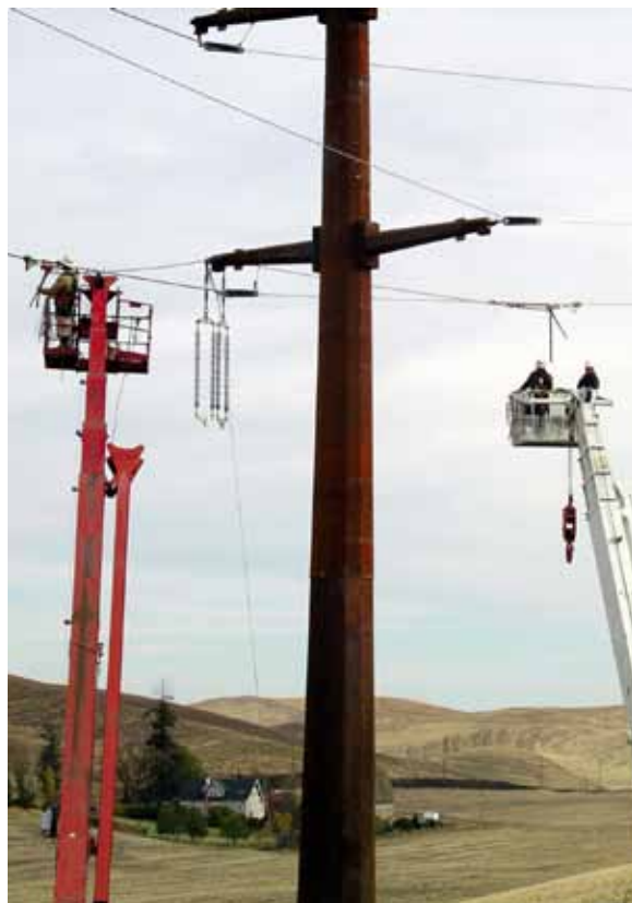
Transmission upgrade work
