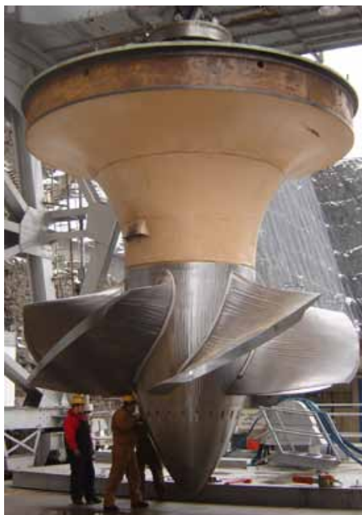
Noxon Rapids turbine upgrade
