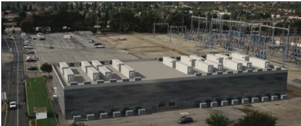
Proposed 100 MW/400 MWh transmission-connected battery.
