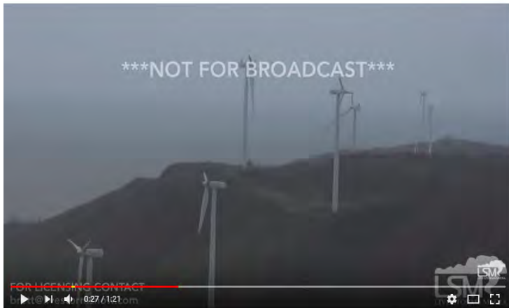
9-22-17 Puerto Rico Wind - Solar - Cellular Structures Destroyed - Aerial
