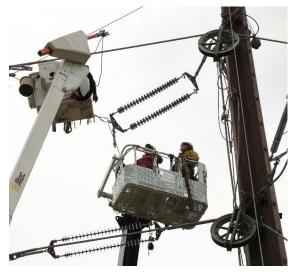
Workers connecting a transmission line to insulators
