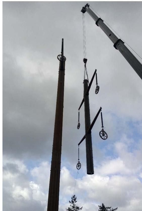
Installing a steel monopole with pulleys attached
