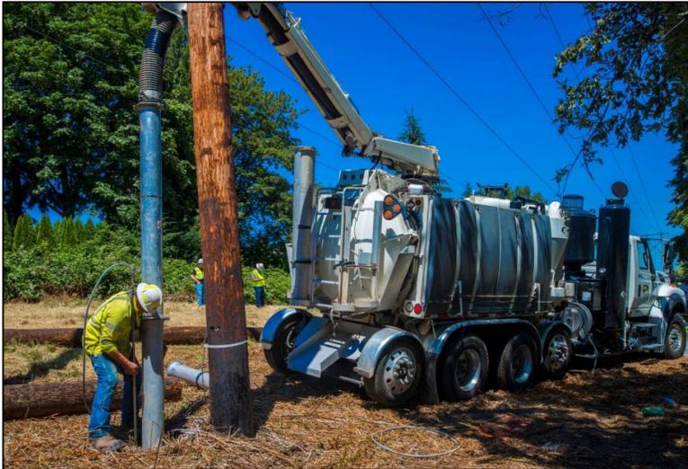
Vacuum truck in the existing corridor in Newcastle excavating a hole for installation of a replacement transmission pole.
