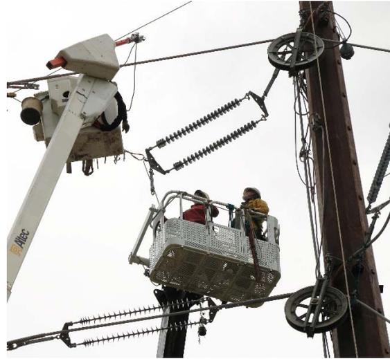
Workers connecting a transmission line to insulators
