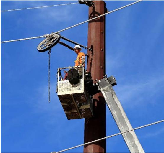
Worker rebuilding a transmission line
