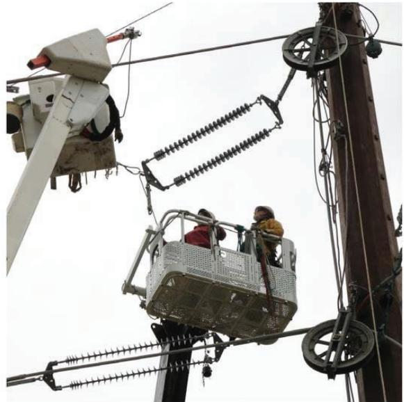
Workers connecting a transmission line to insulators
