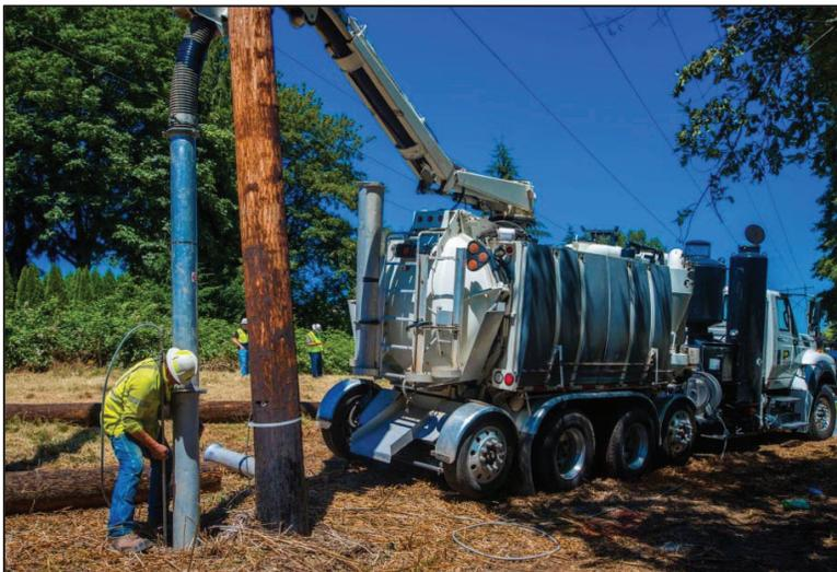
Vacuum truck in the existing corridor in the Newcastle segment excavating a hole for installation of a transmission pole.
