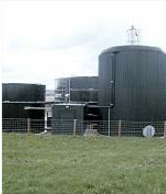
Figure 2-18. Anaerobic Digester (Biomass Energy Centre, 2015)
