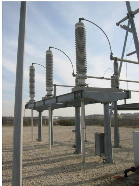
**Figure 2-13 Typical HPFF Terminations in a Substation**
