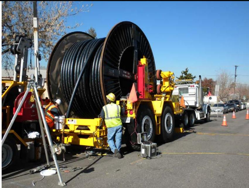
Figure 2-10 Typical Cable Pulling Set up
