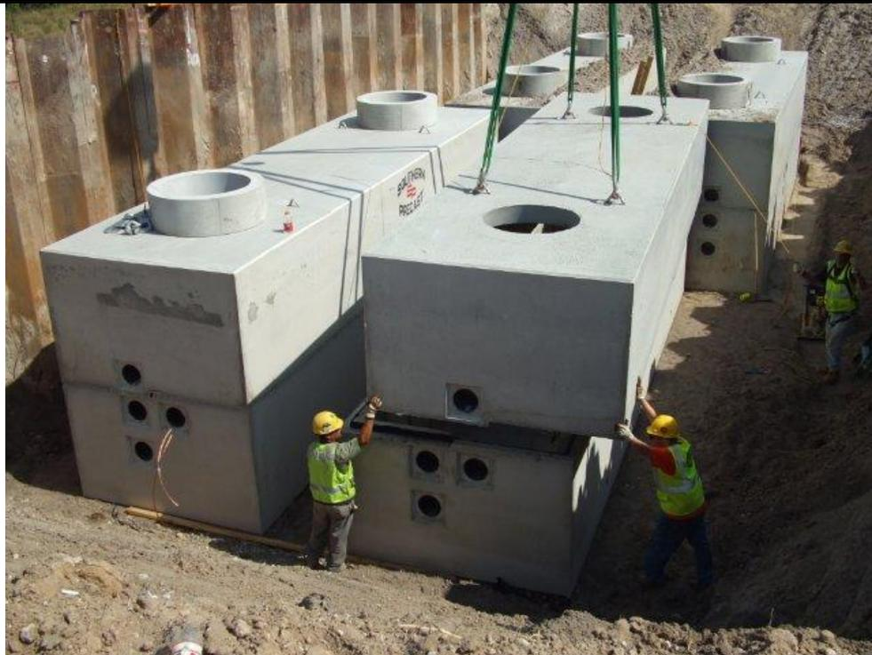
**Figure 2-9 Splicing Vault Installation**
