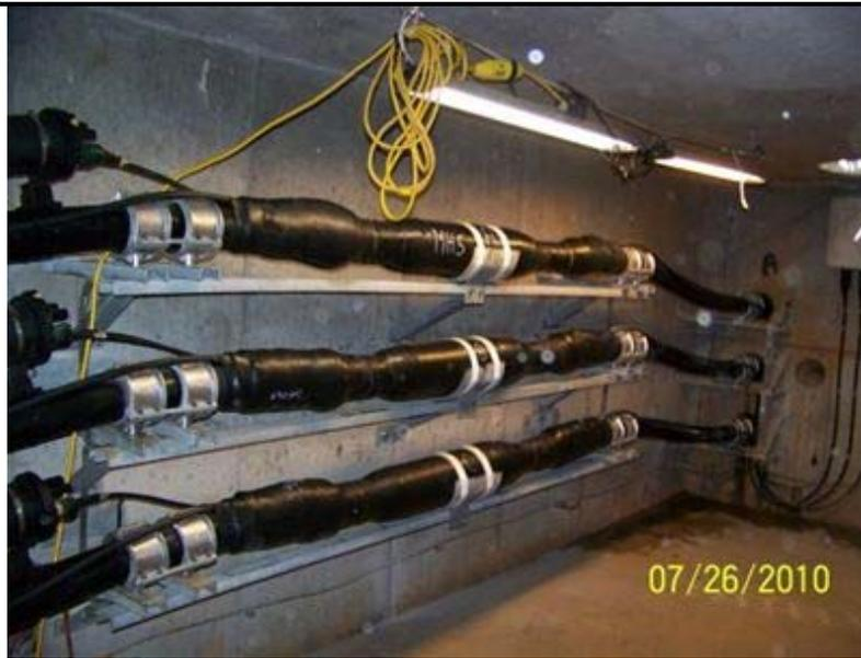
**Figure 2-2 Typical 230 kV Pre-Molded XLPE Splices**
