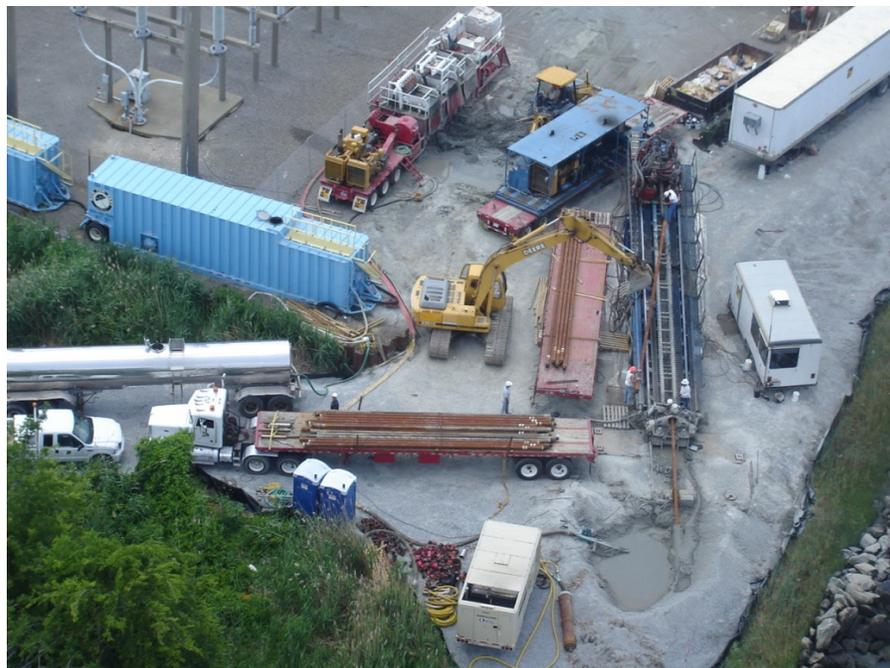
Figure 2-7 Typical HDD Setup
