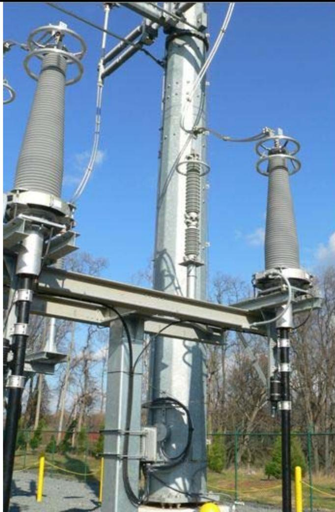
Figure 2-3 Typical 230 kV XLPE Terminations
