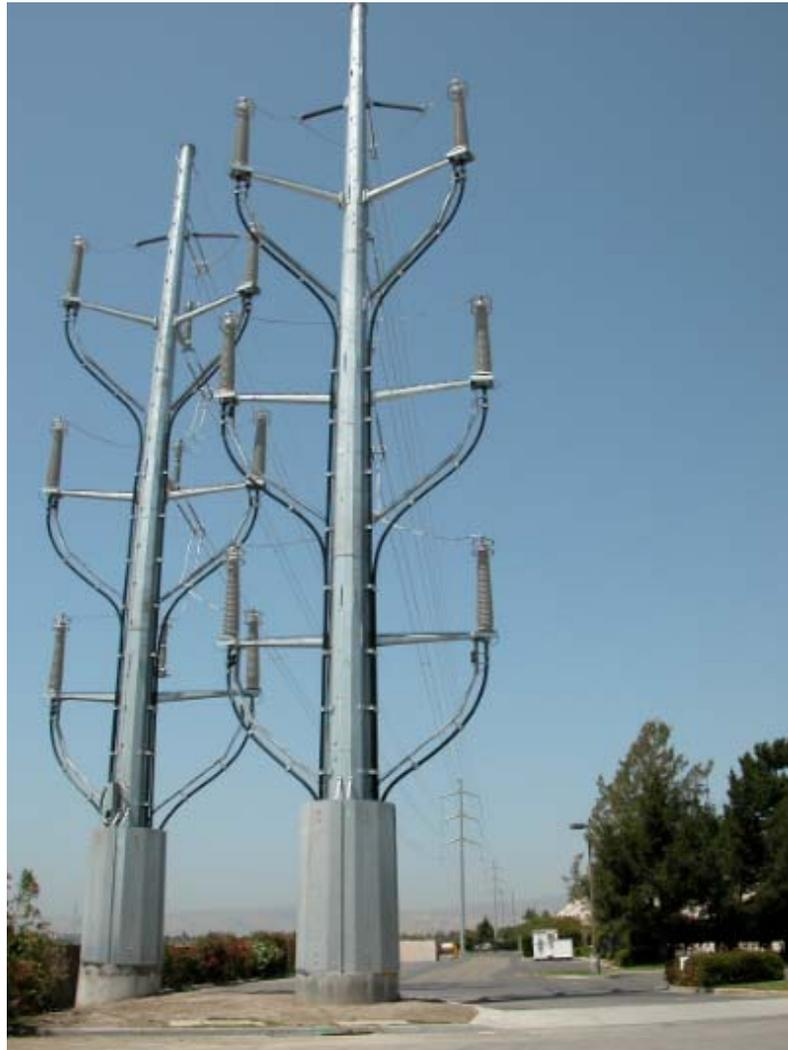
**Figure 3-10 Typical 230 kV Riser Structure**
