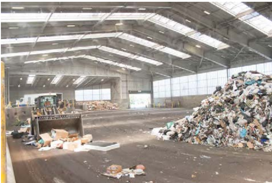
Bow Lake Recycling and Transfer Station
