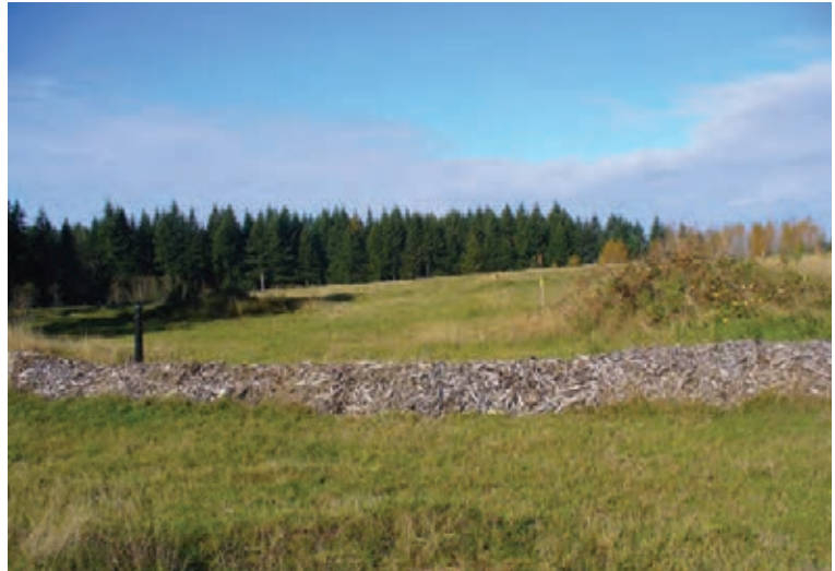
A bioberm at the Cedar Falls closed landfill filters landfill gas.
