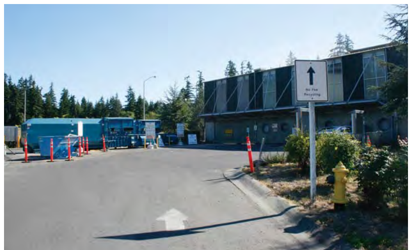
The Vashon Recycling and Transfer Station
