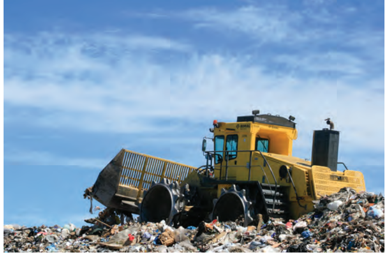
Heavy equipment compacts garbage in place at Cedar Hills.
