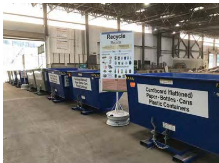
The new Factoria Recycling and Transfer Station has two compactors and room for an recyclables collection
