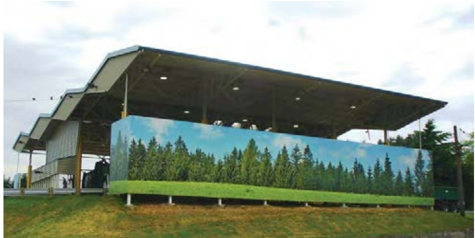
The Houghton Transfer Station
