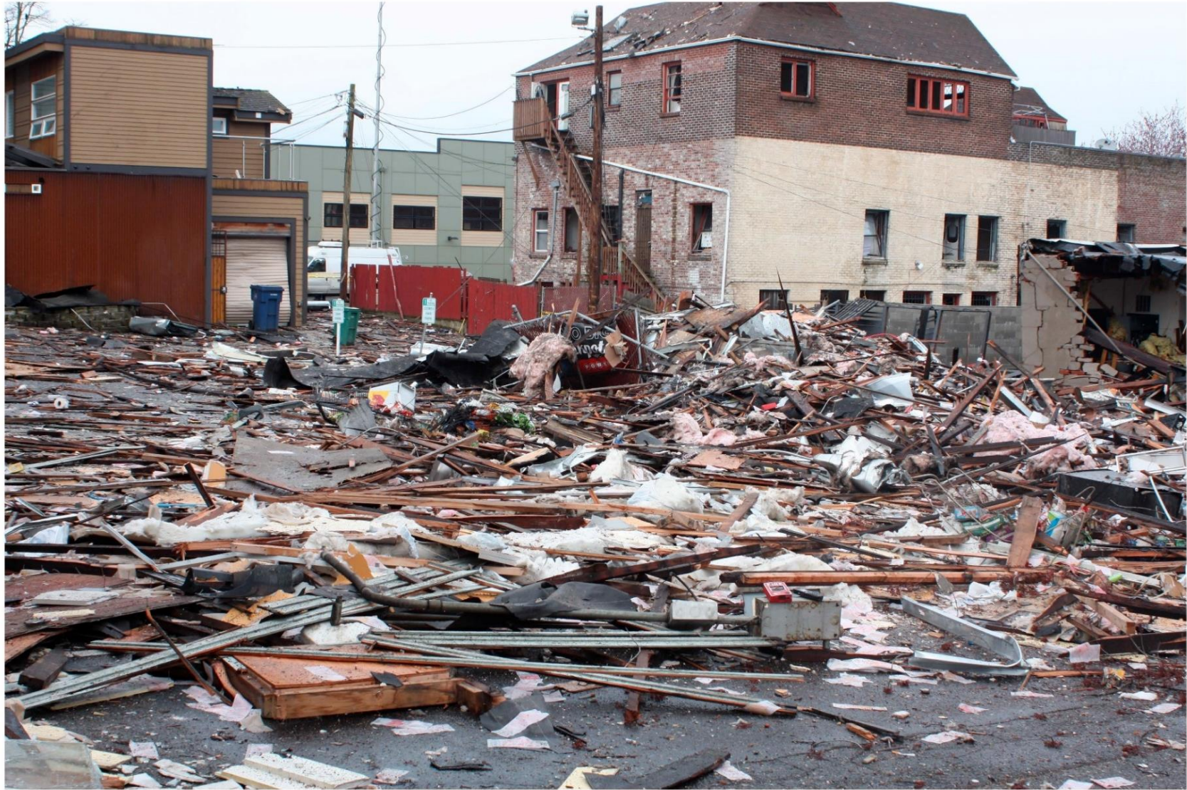
Image 3. Debris spread facing west from Greenwood Avenue North.
