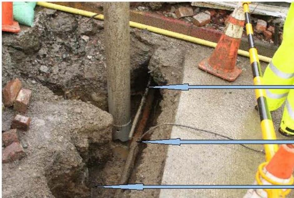
Image 12. Illustration and image depicting excavation of service line and foreign line post-incident.
