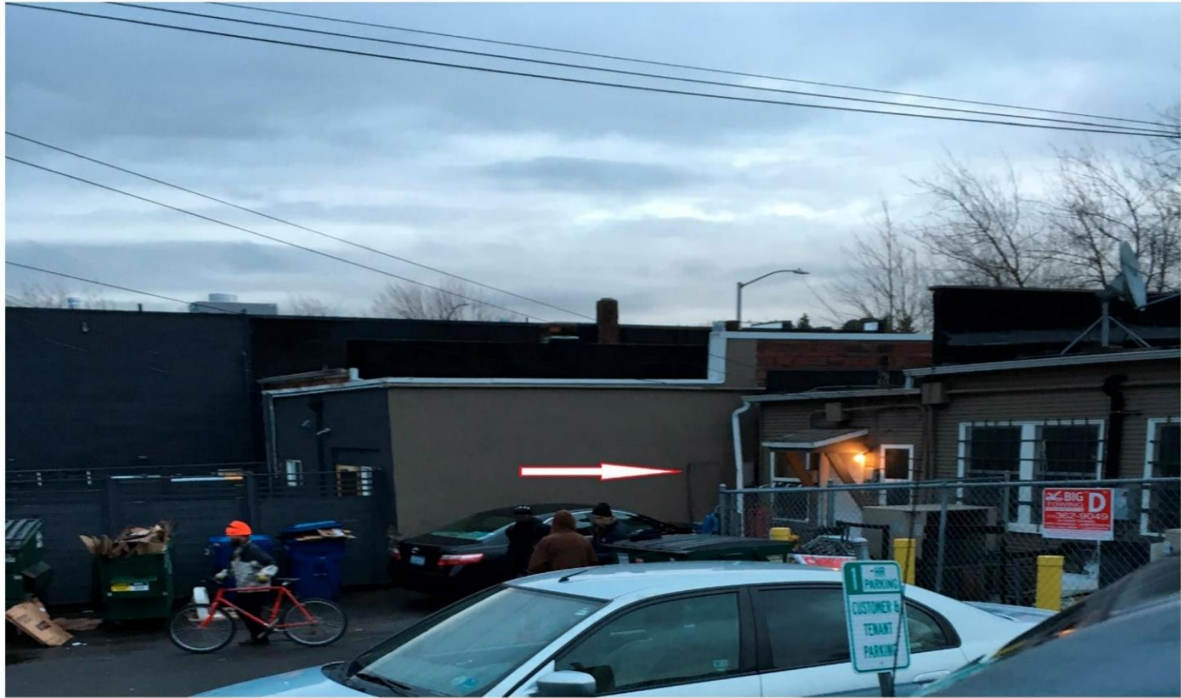
Image 9. Location of narrow space between Mr. Gyros and Neptune Coffee buildings where leak occurred.
