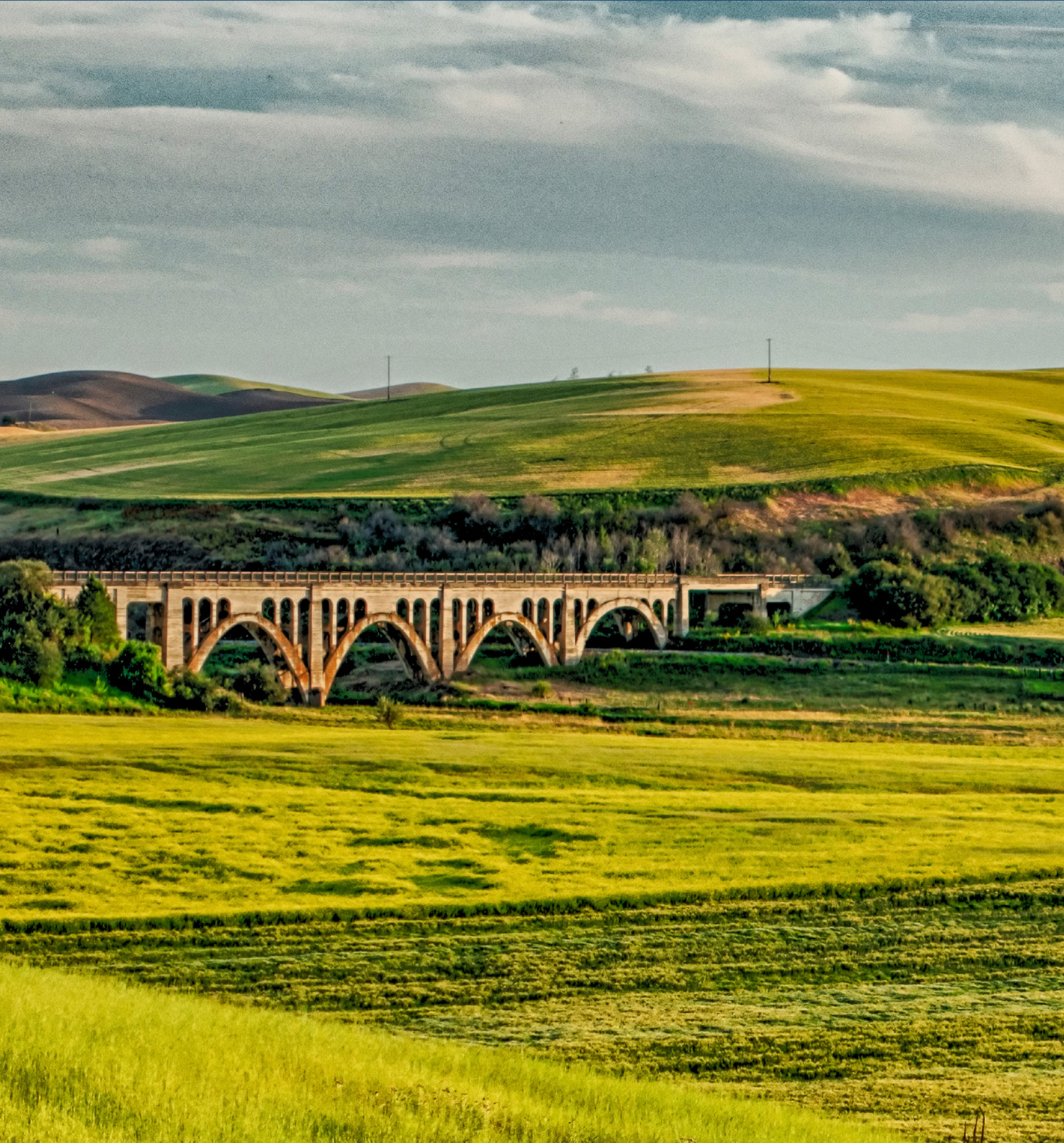
Milwaukee Road Railroad Bridge, Rosalia, Washington
