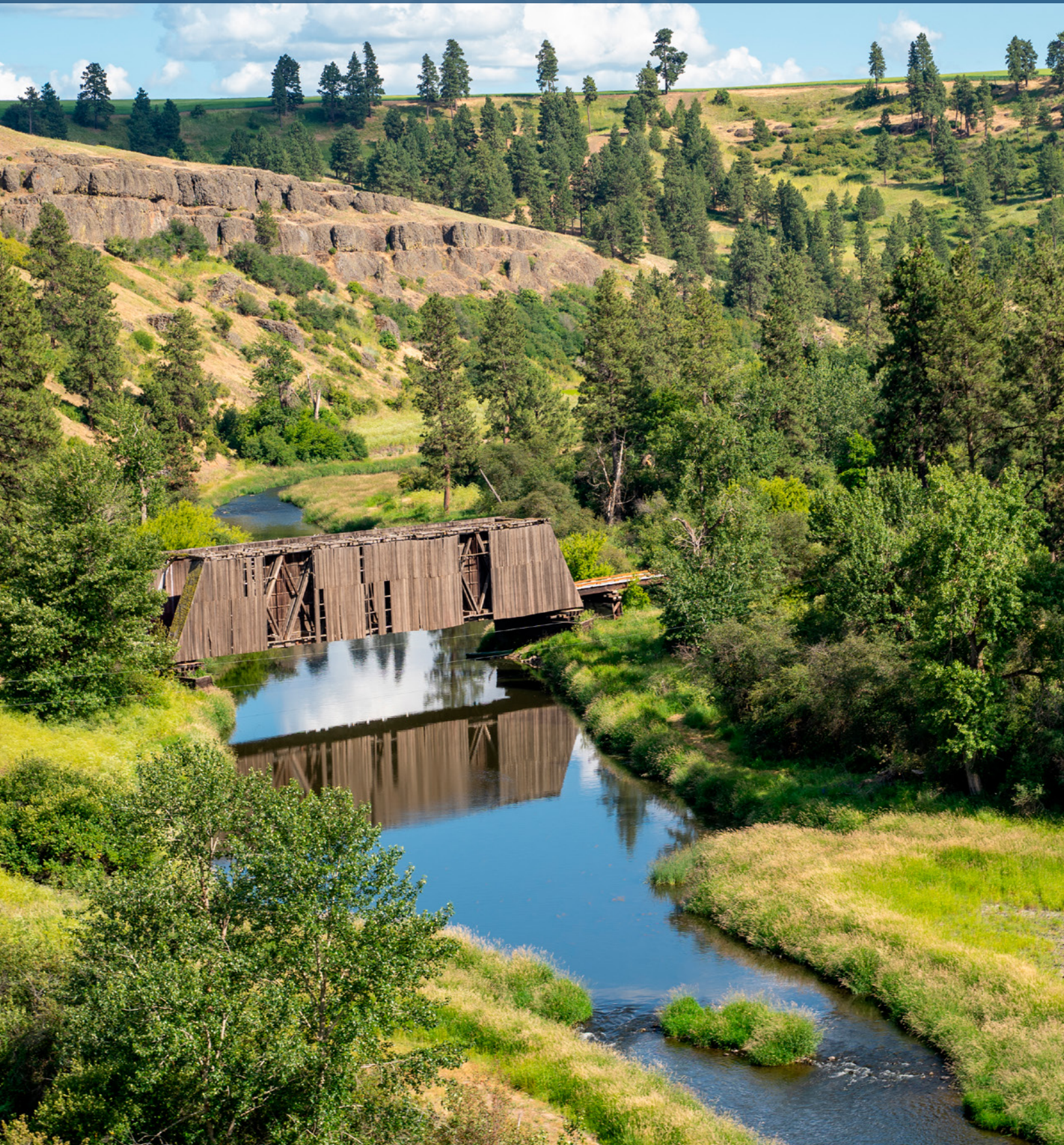
Manning-Rye Covered Bridge, Colfax, Washington
