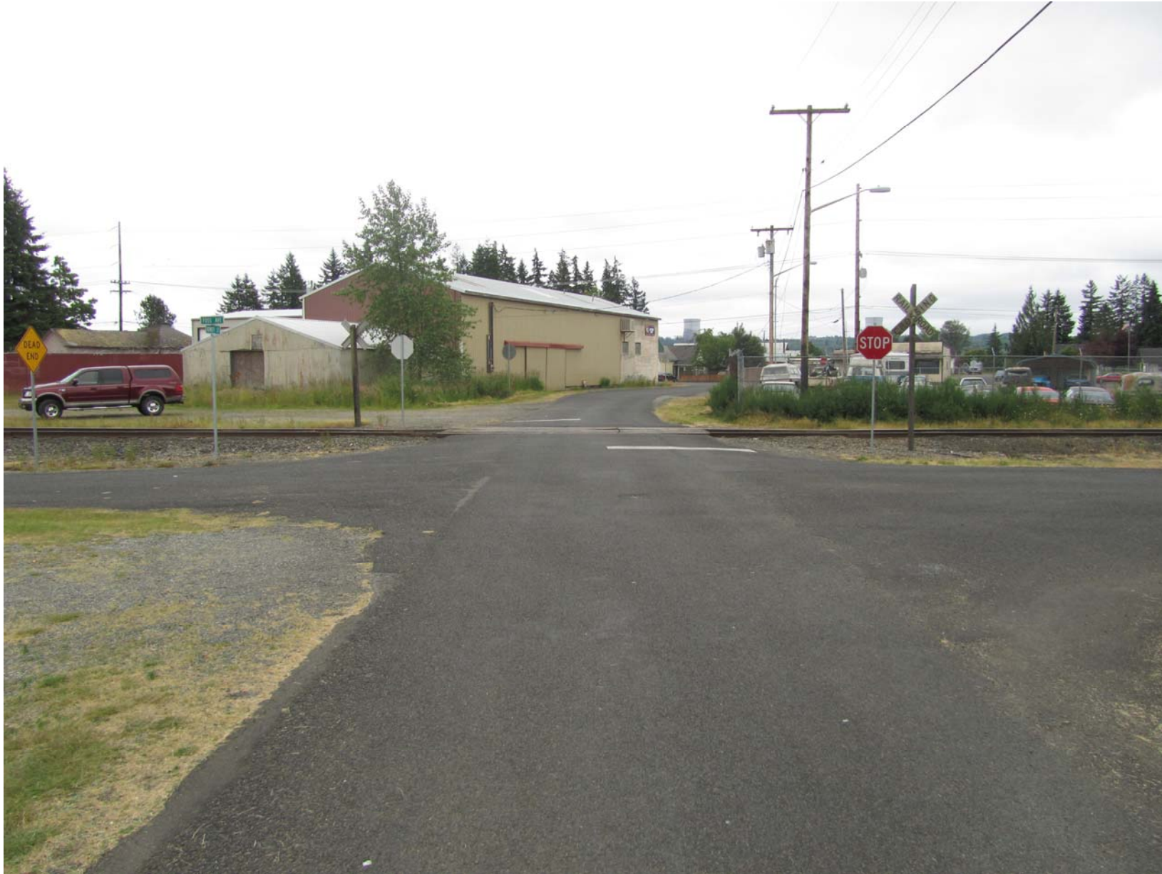
View looking south at Hewitt Street crossing, Satsop, Grays Harbor County
