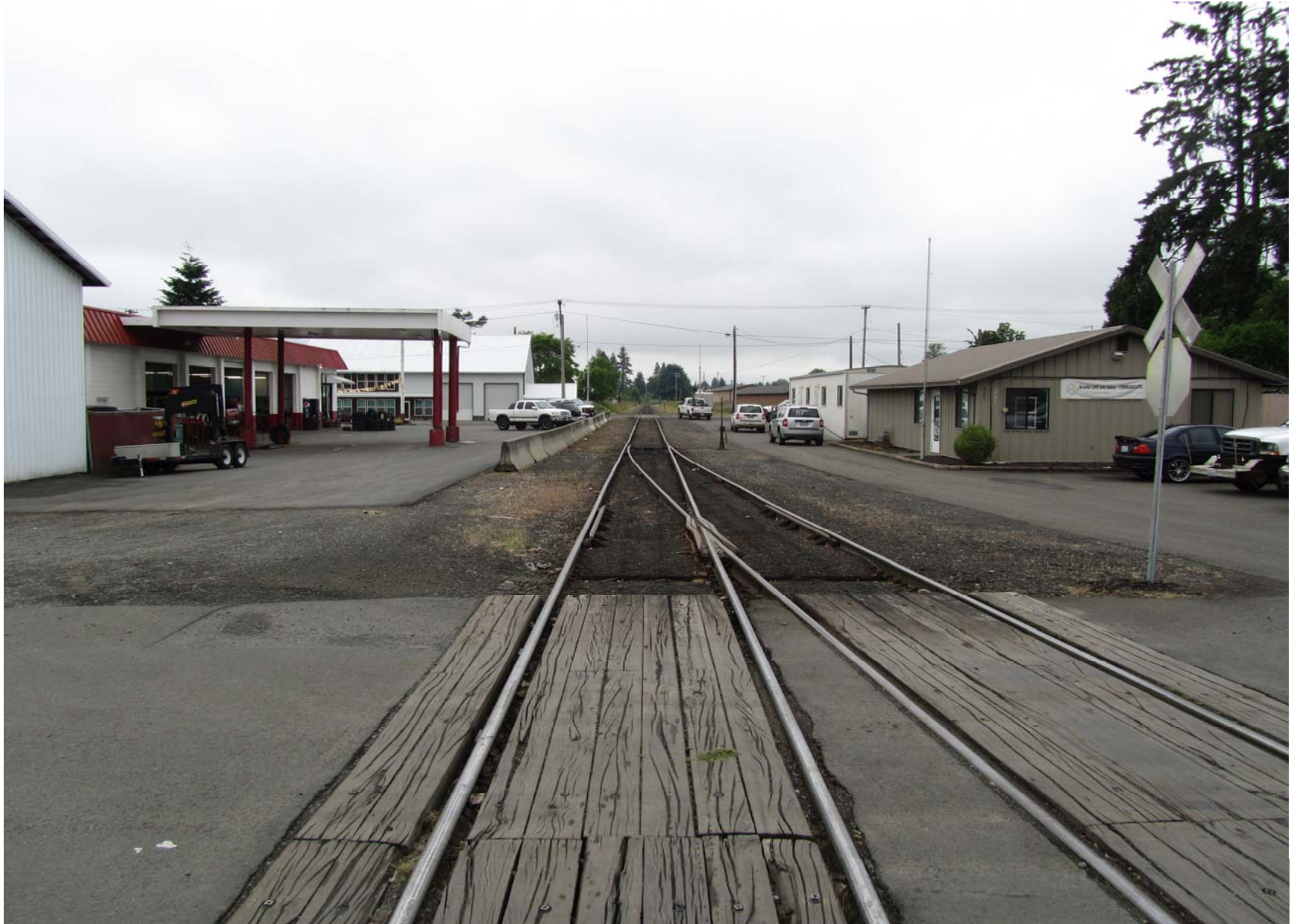
View looking west standing at the N. 2 nd Street crossing, Elma
