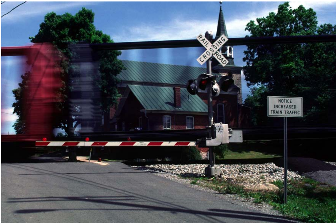
A freight train becomes a blur as it passes through a grade crossing that has flashing lights, fully activated gates, and a warning sign to the right.
