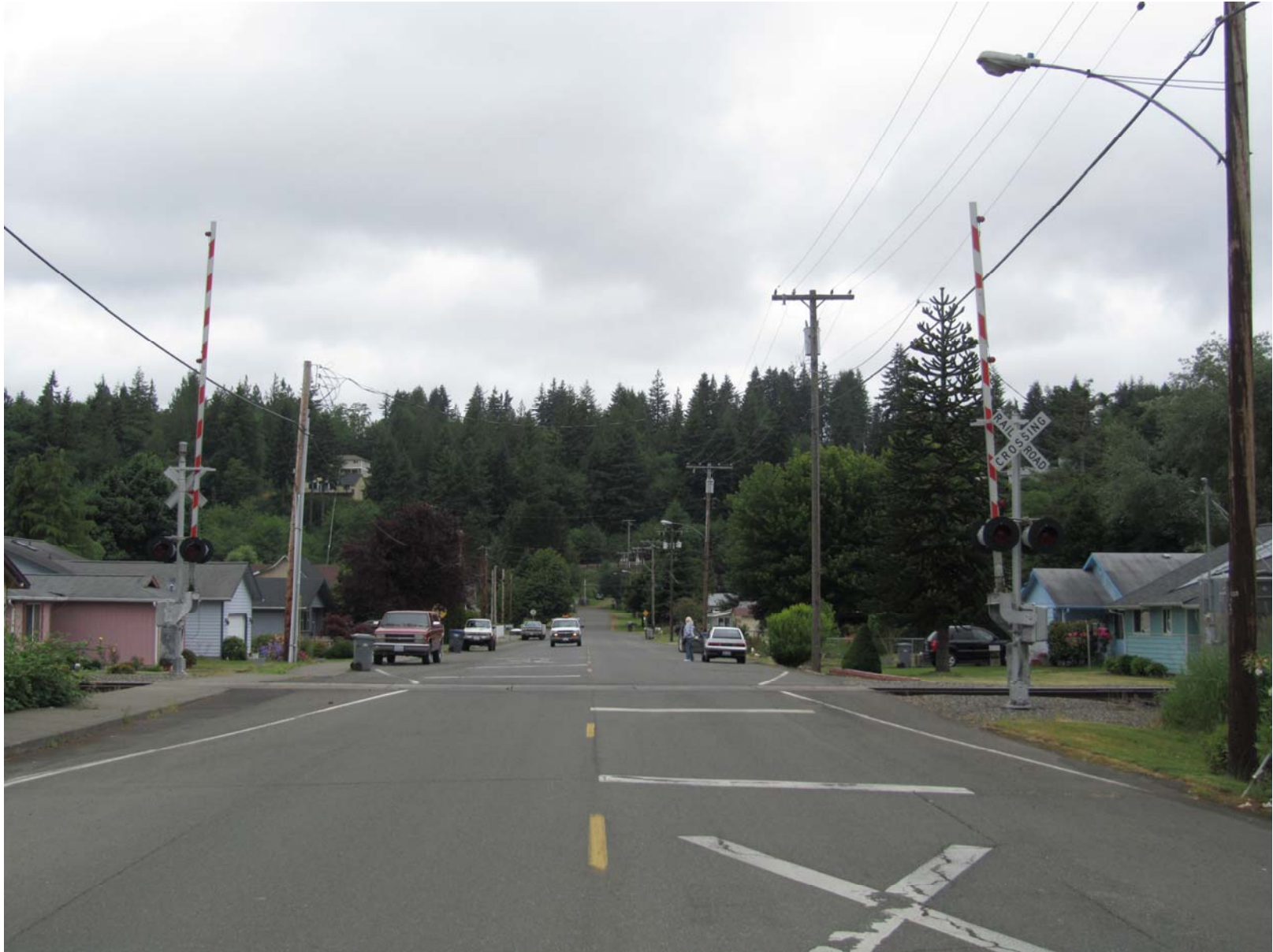
View looking north at the N. 11 th Street Crossing, Elma
