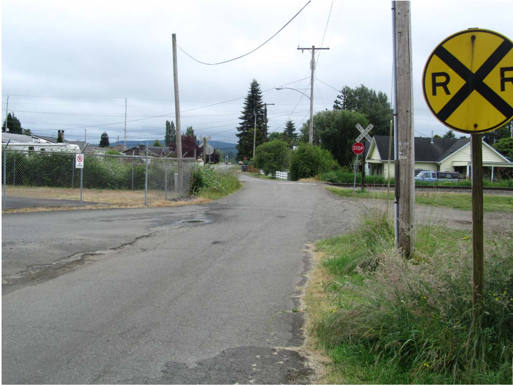
View looking south towards the N. 6 th Street crossing, Elma
