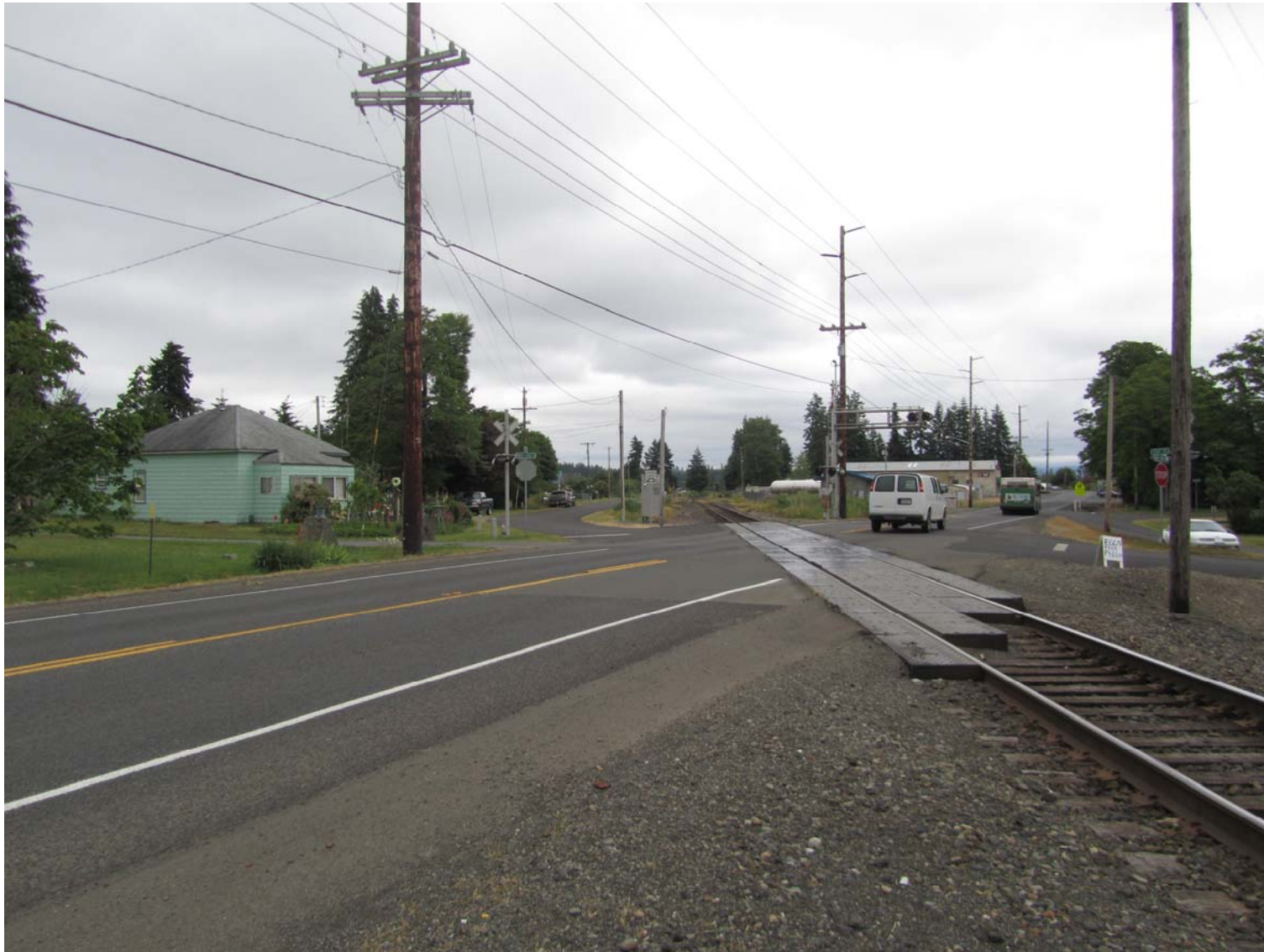
VIEW AT FOSS/ASH STREET CROSSING LOOKING EAST DOWN MONTE/ELMA HIGHWAY
