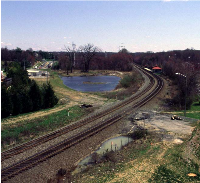
A two-track mainline railroad passes through a recently removed grade crossing.
