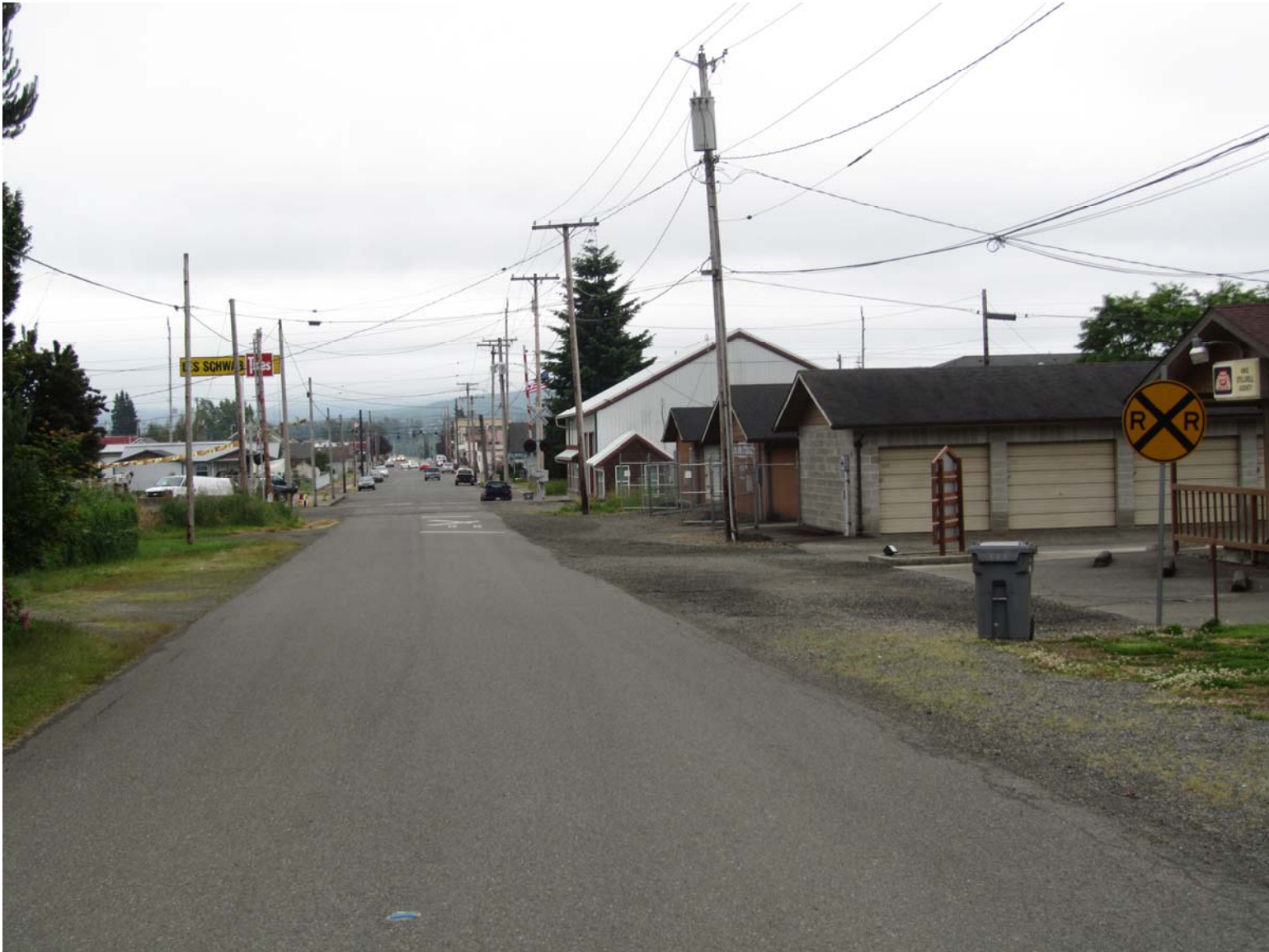
View looking south towards the N. 3 rd Street crossing, Elma
