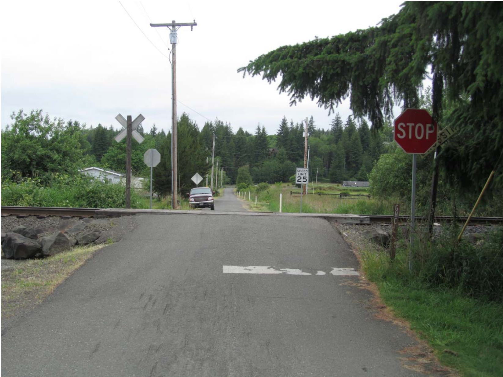
View looking north at the N. 17 th Street crossing, Elma
