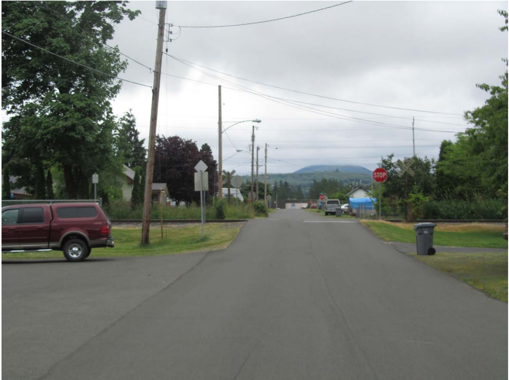
View looking south towards the N. 10 th Street crossing, Elma
