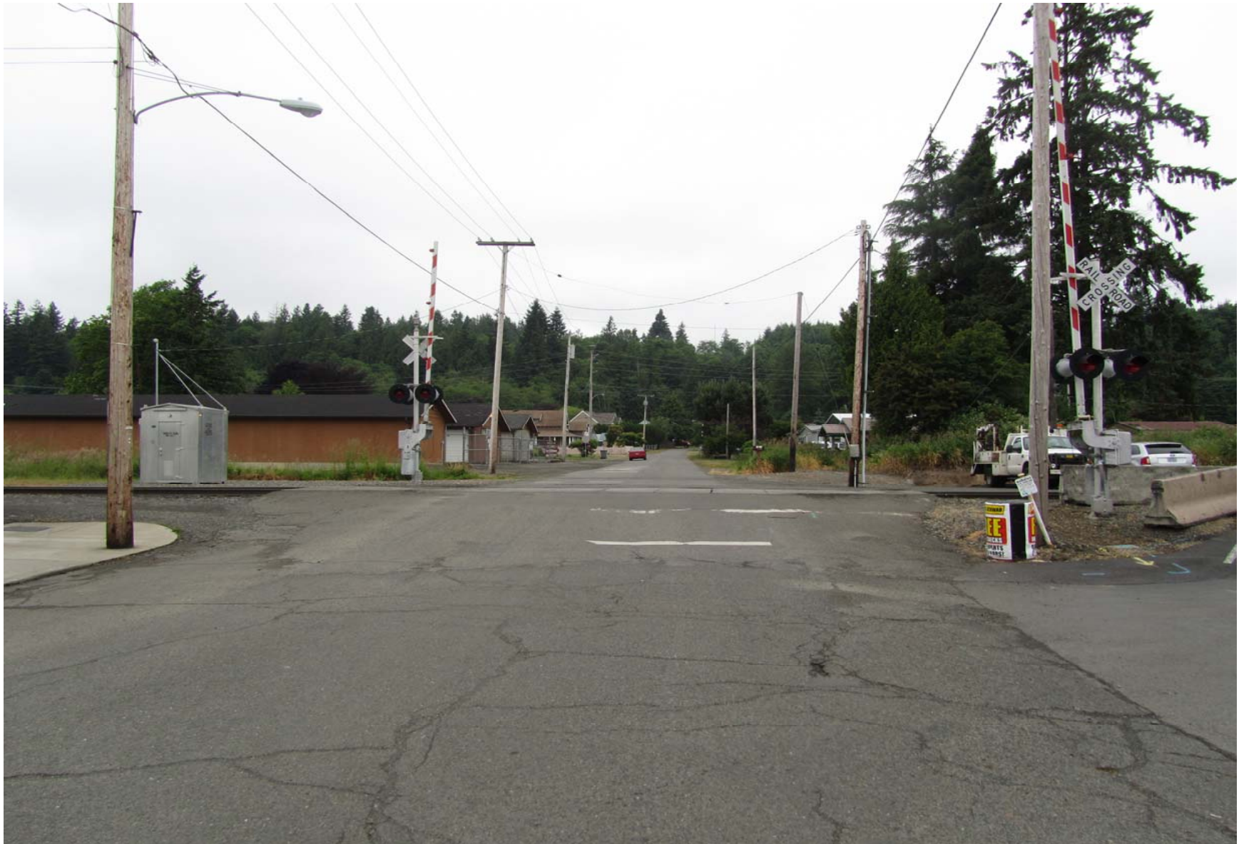
View looking north at the N. 3 rd Street crossing, Elma
