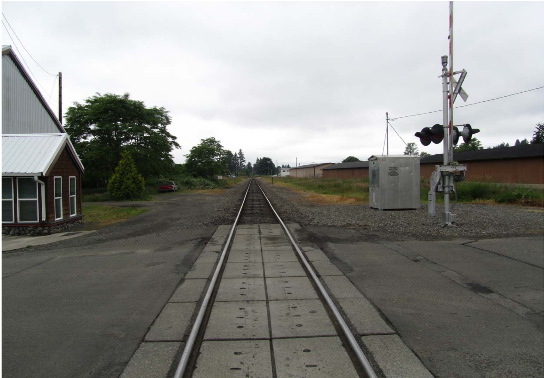
View looking west at the N. 3 rd Street crossing, Elma
