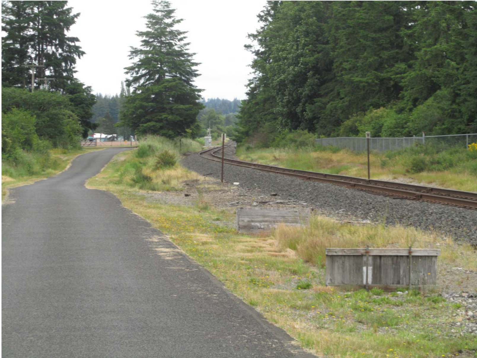
View looking east at Hewitt Street crossing, Satsop, Grays Harbor County
