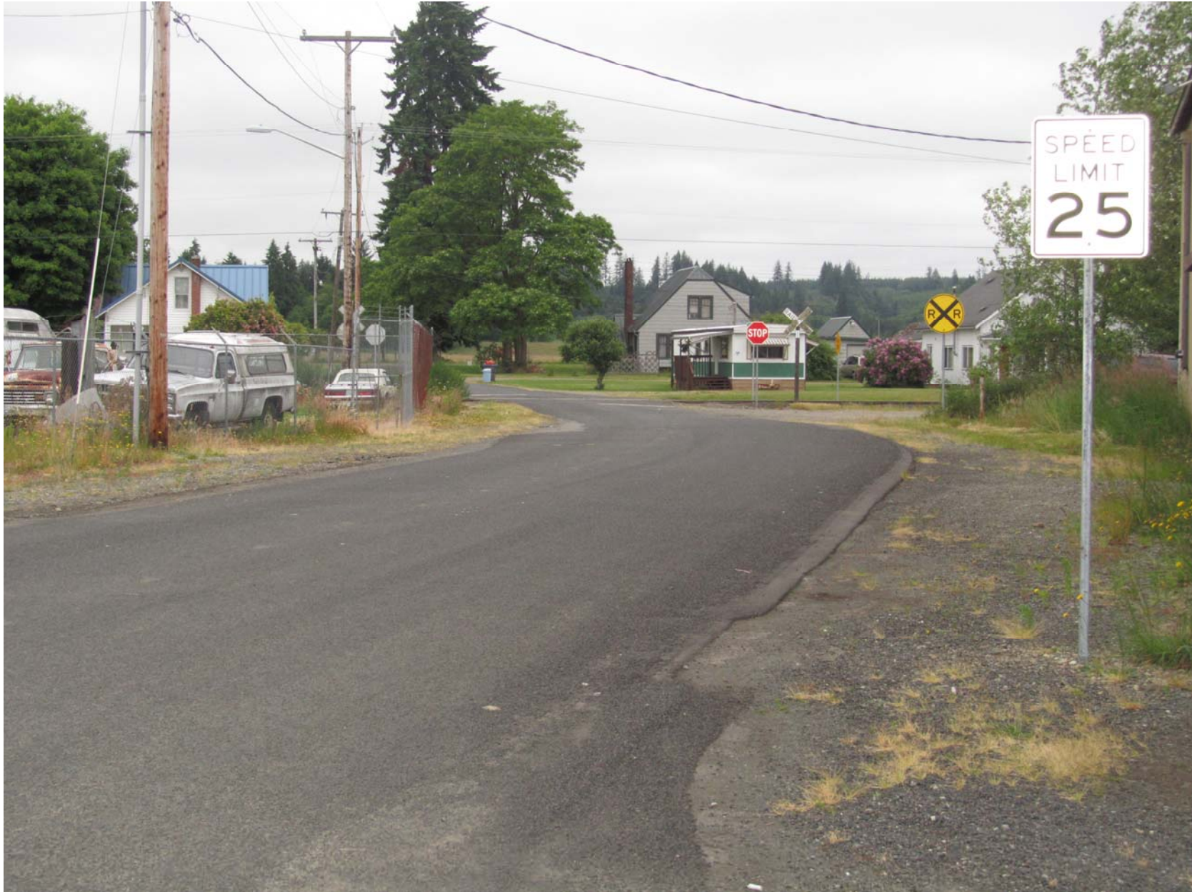
View looking north at Hewitt Street crossing, Satsop, Grays Harbor County
