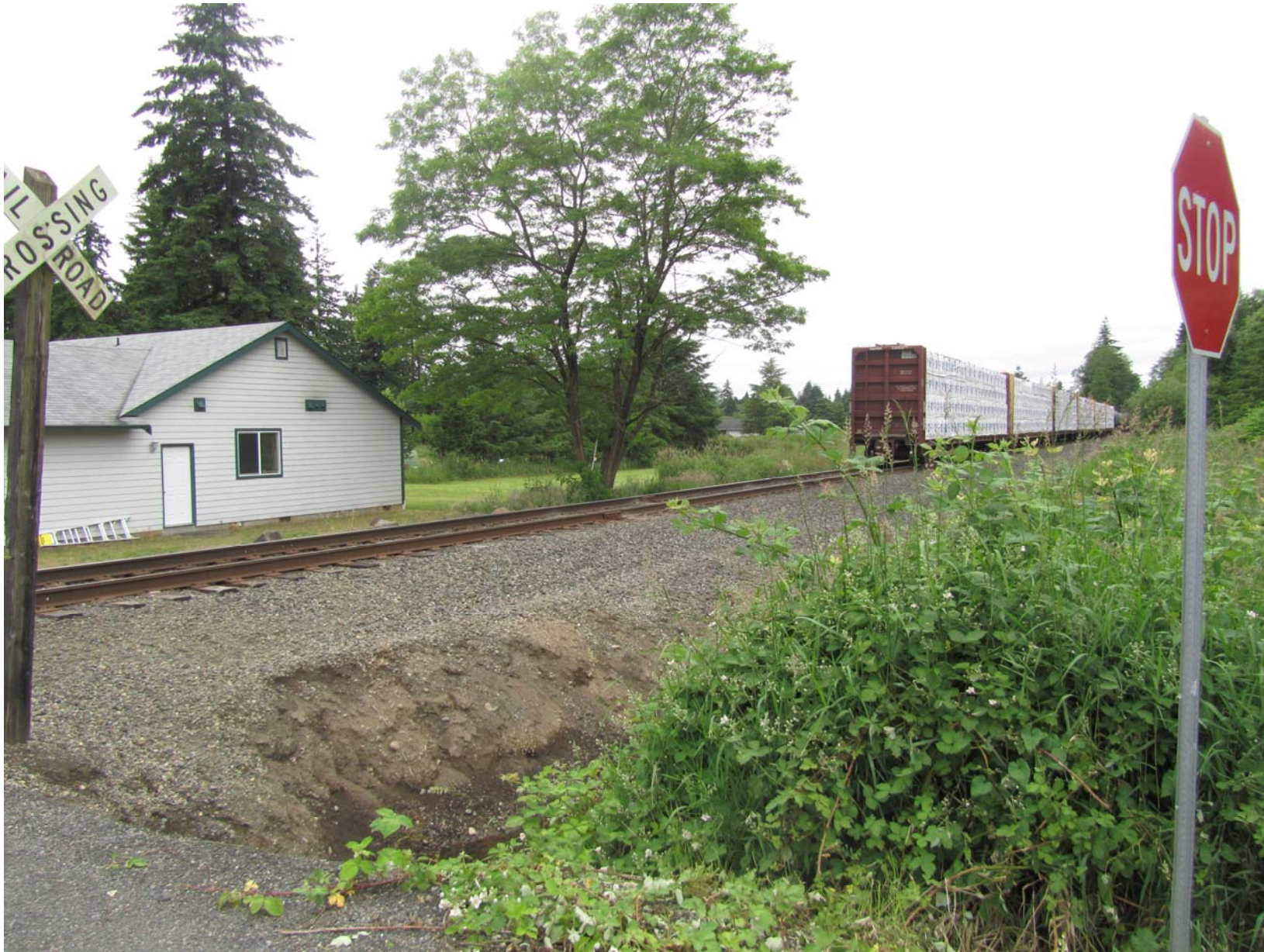
View looking west at the N. 17 th Street crossing, Grays Harbor County
