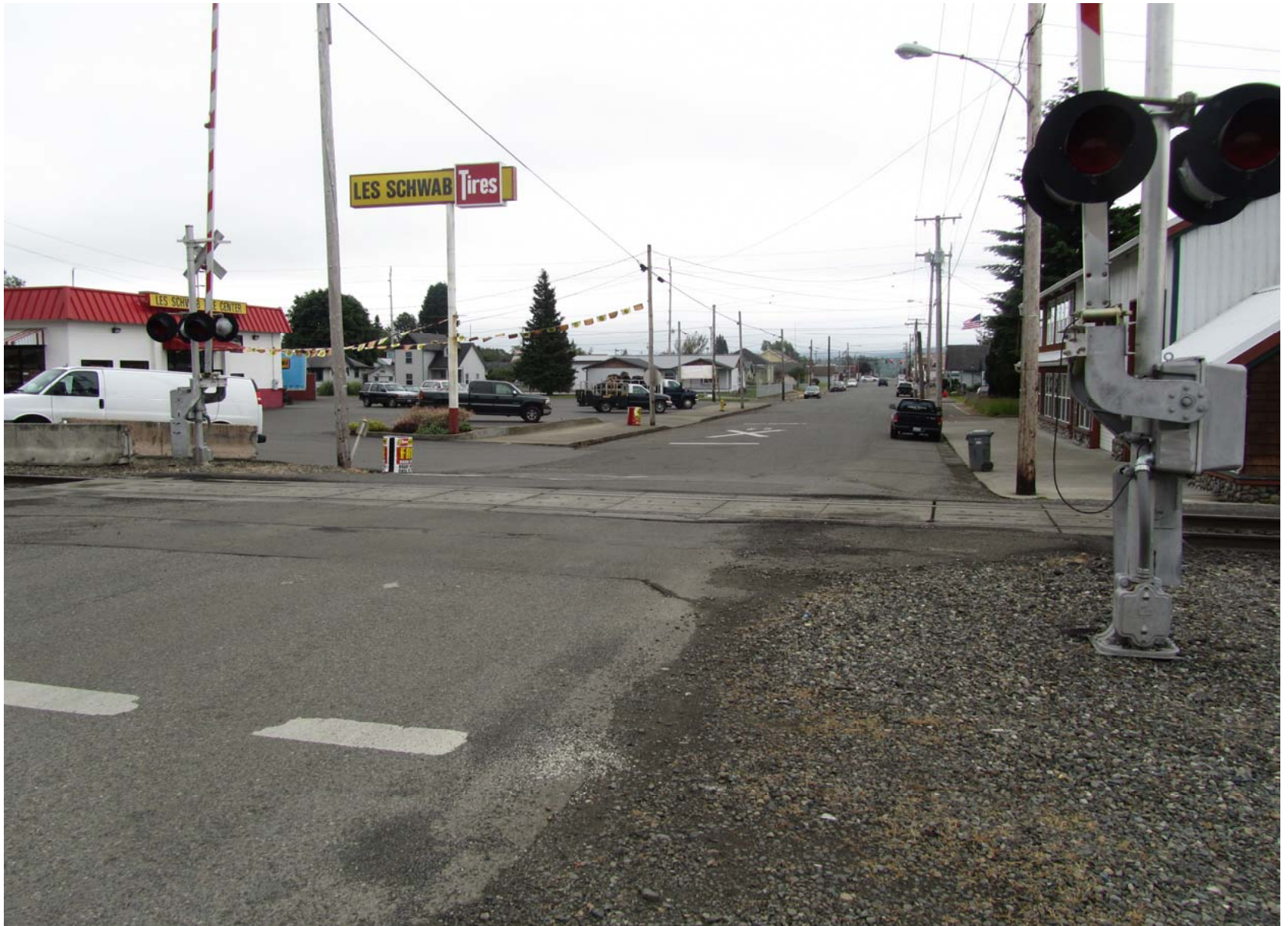
View looking south at the N. 3 rd Street crossing, Elma
