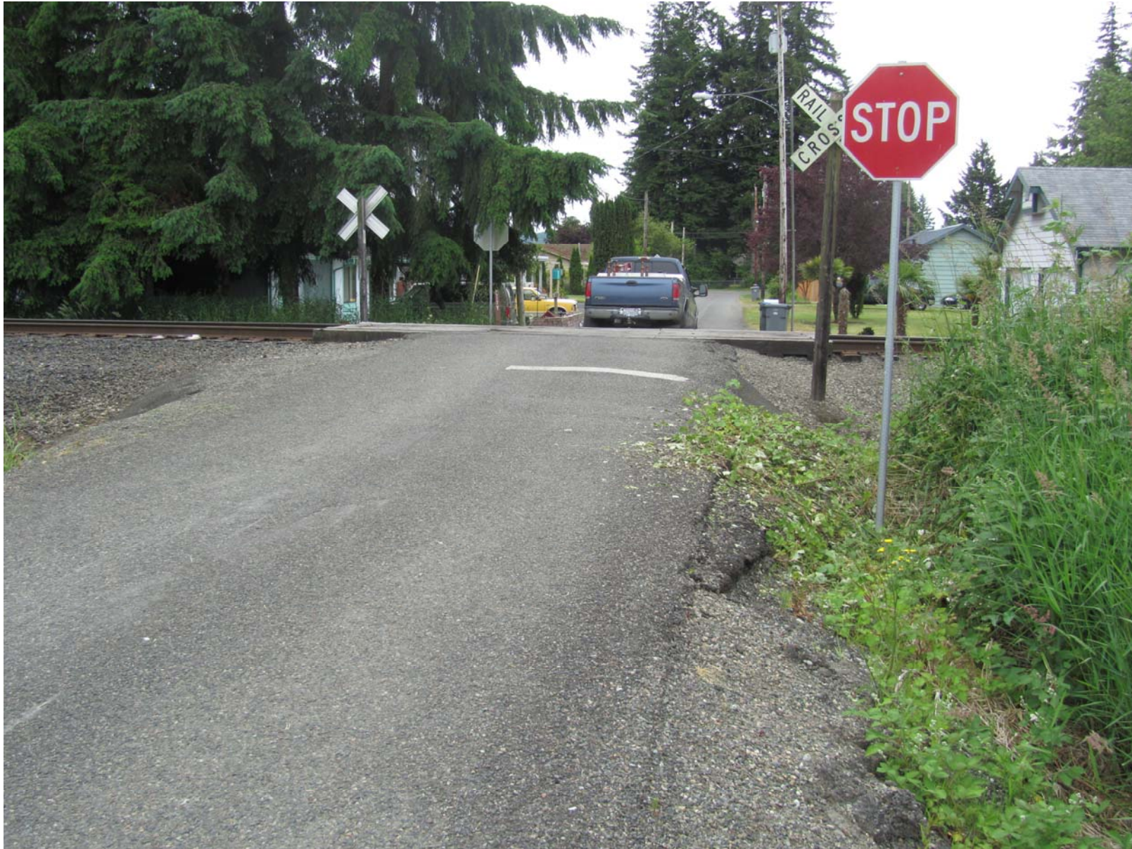
View looking south at the N. 17 th Street crossing, Grays Harbor County
