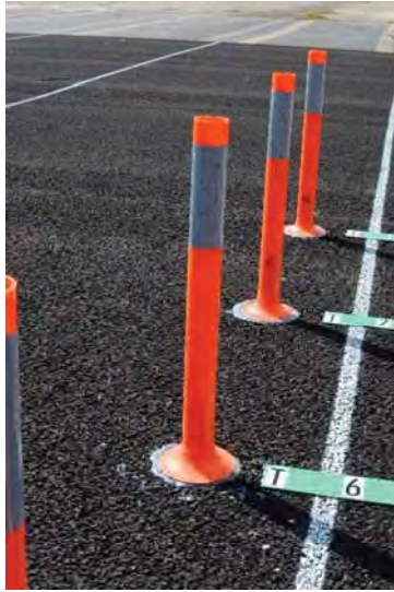
Figure 3.54. 607531-02-4 Sample (Asphalt Surface).
