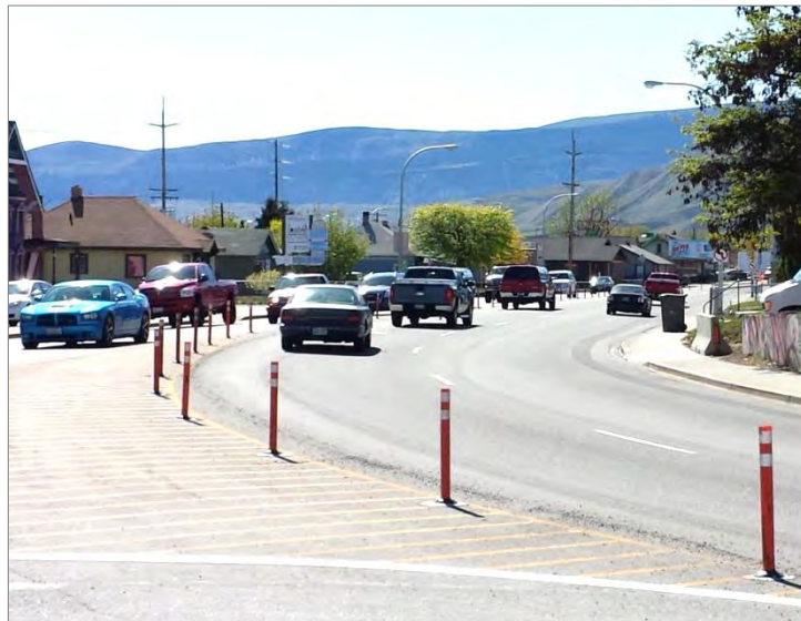
The City of Wenatchee has modified the Chelan Avenue connection with Mission Street to reduce the impacts of off-tracking of large trucks.
