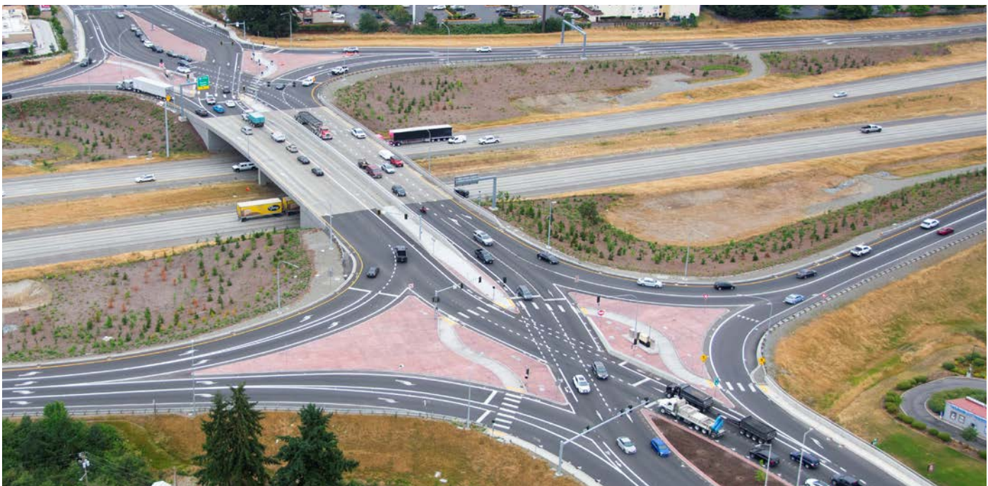
The diverging diamond at SR 510 and Interstate 5 in Lacey is the first of its kind in Washington state. And not only improves traffic flow across the busy intersection but reduces the potential for crashes.
