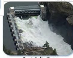
Post Falls Dam
