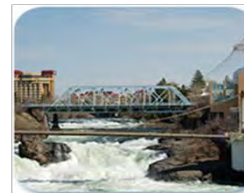
Upper Falls Dam
