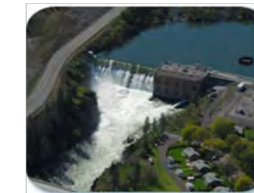
Nine Mile Dam
