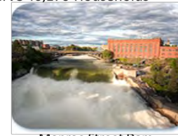
Monroe Street Dam
