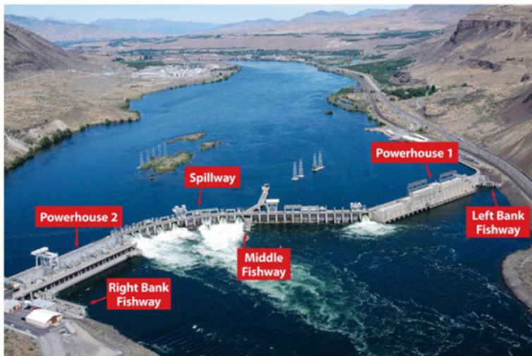
Figure 3: Rock Island Hydroelectric Project
