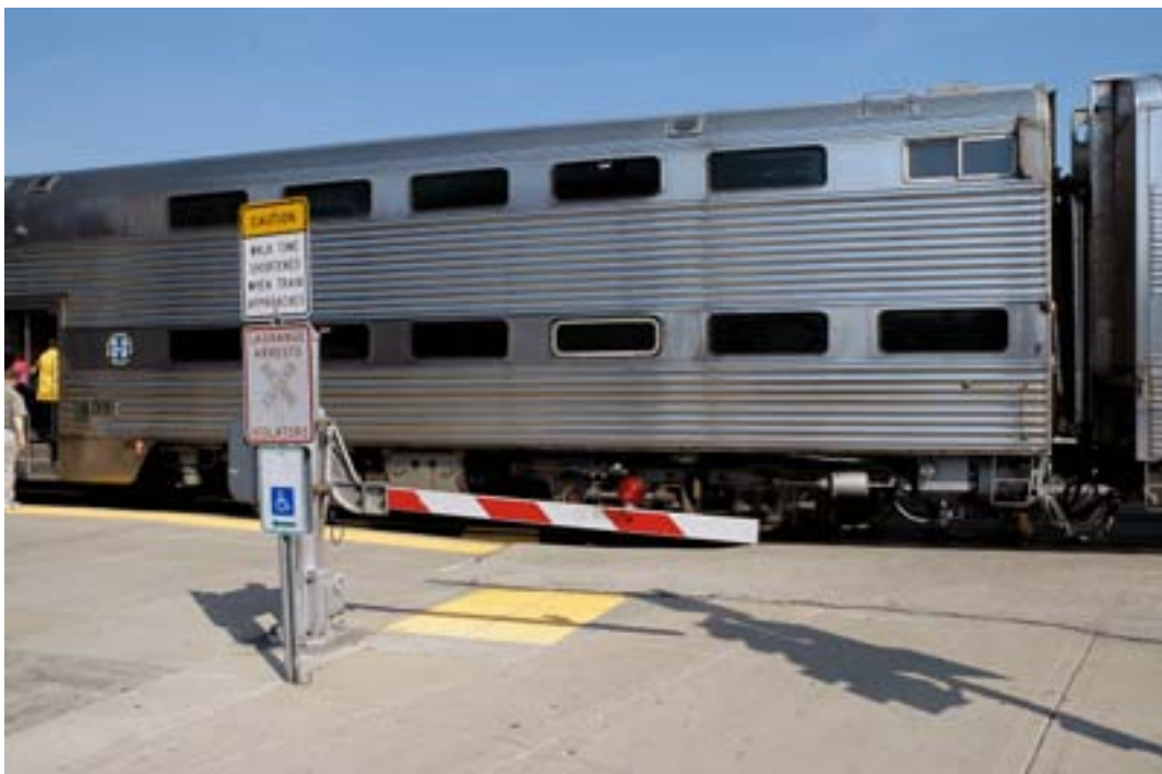
Stone Avenue Metra station (ABOVE) in LaGrange, IL features these pedestrian warning devices between inbound and outbound platforms. Short gate arms (BELOW) are used at the LaGrange Road station.
