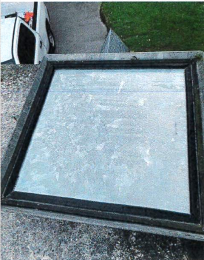
New reservoir hatch seal
