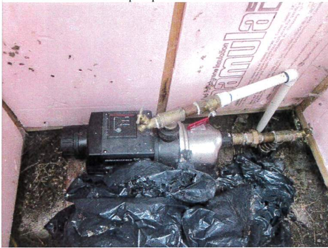
Booster pump enclosure
