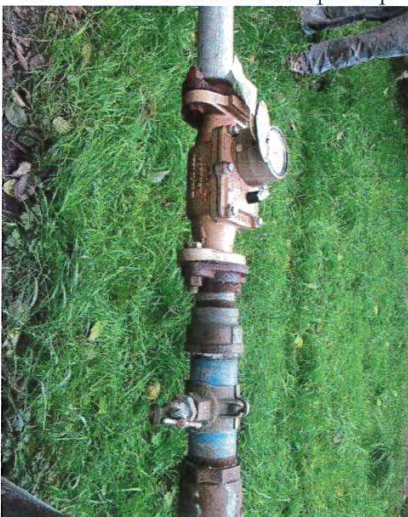
SO3 water meter and sample tap
