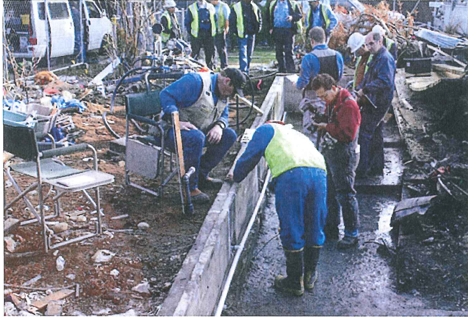
Photo 11: View of the east foundation wall (looking south) and the crawlspace concrete floor (right of the wall). The white plastic pipe at the base of the wall was supplied for use in the test. Photo taken November 8, 2011, by Scott Rukke, UTC engineer.
