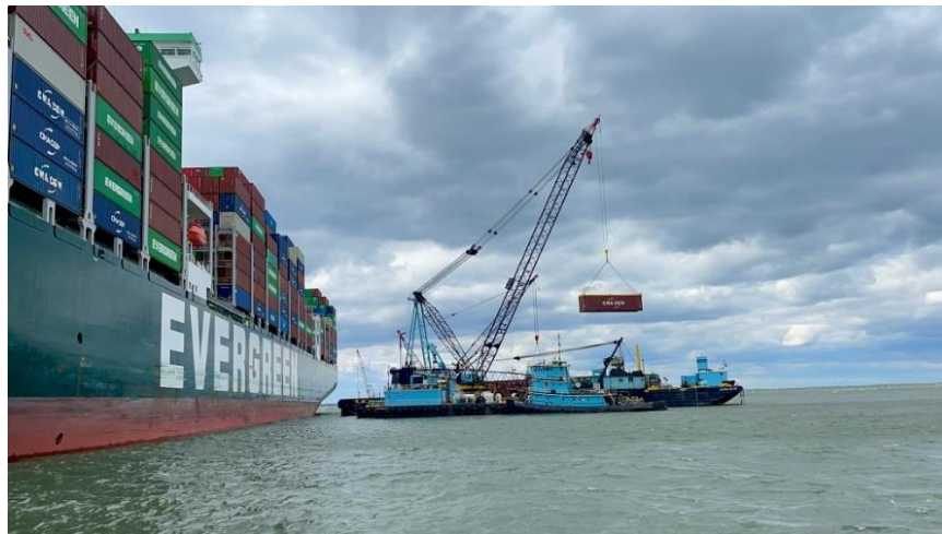
Figure 11. Crane operations on the port side of the EVER FORWARD during attempts to refloat the vessel. This photograph was provided by USCG District 5 Public Affairs.
