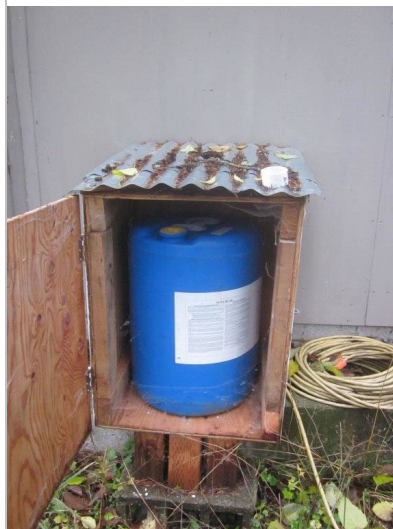
Chlorine solution storage
