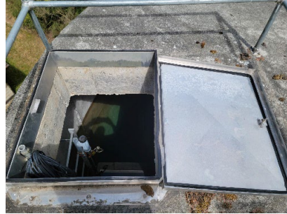
Tank 3 hatch & gasket
