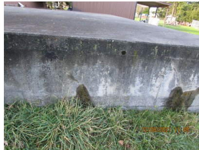
East Side Large Storage Tank
