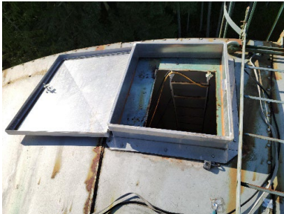
Tank 2 hatch & gasket
