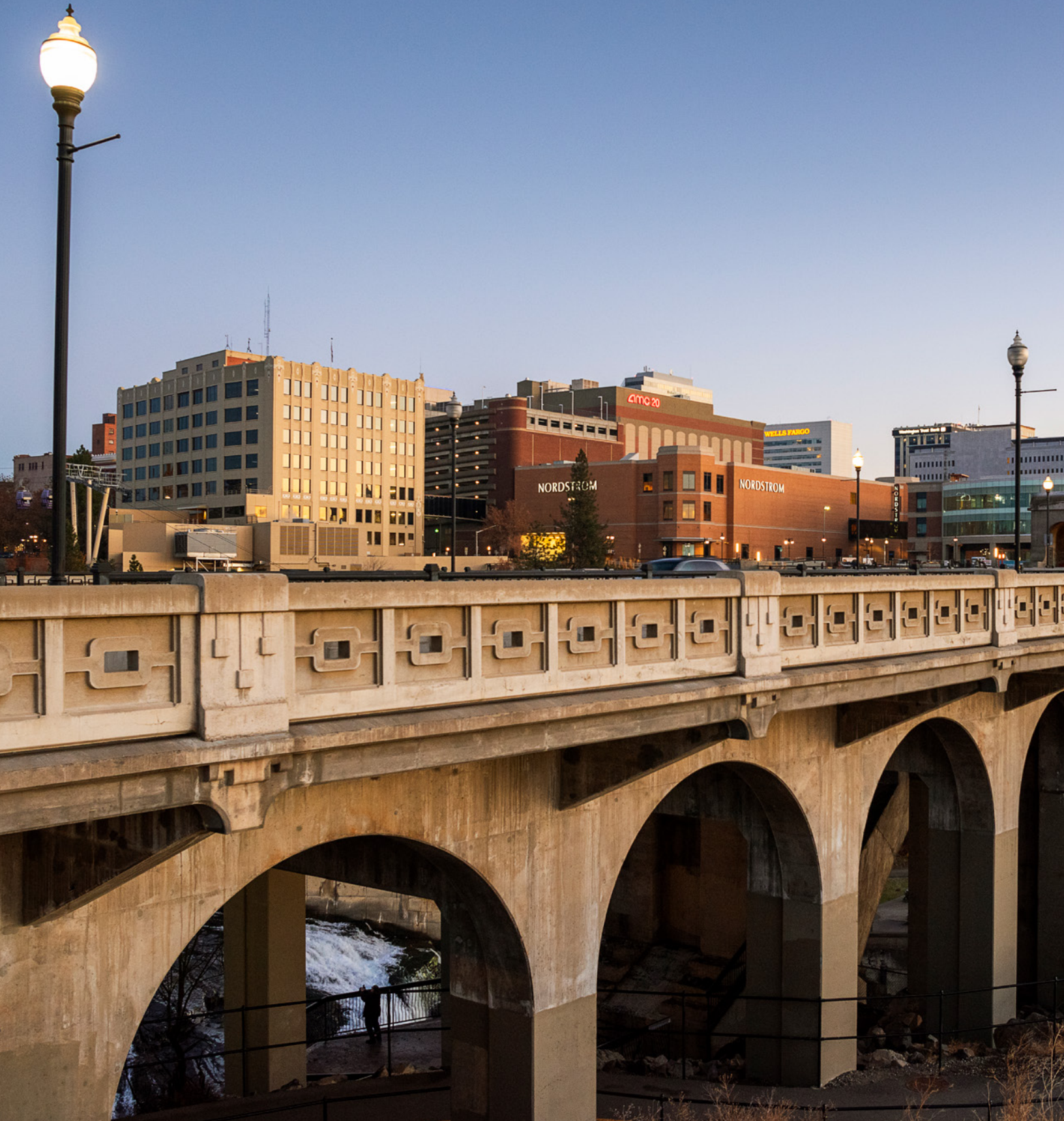
Monroe Street Bridge, Spokane, Washington
