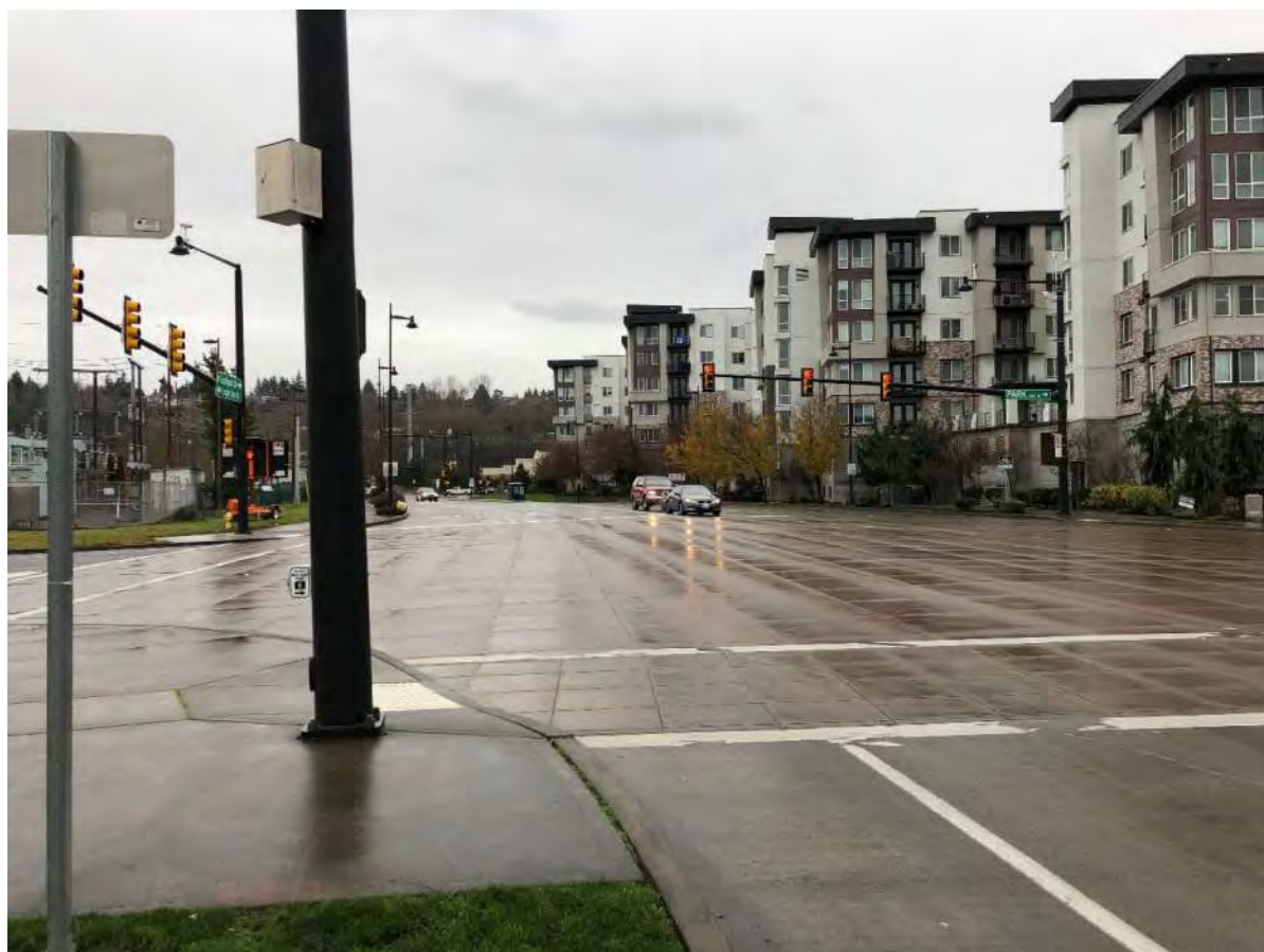
Logan Avenue – Looking East Towards Park Avenue/Southport Drive Intersection
