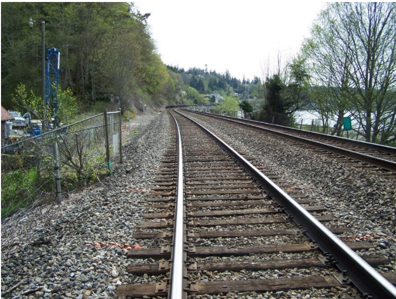
Photo 4 – Main 1 and Main 2 Tracks above the culvert and embankment (existing)
