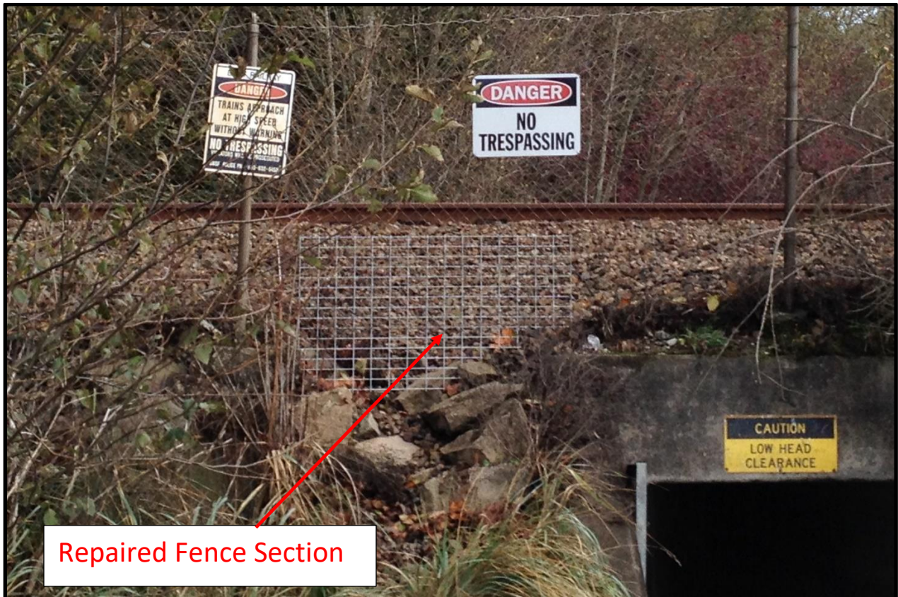
Photo 10. Repaired fence section (downstream/beach side)
