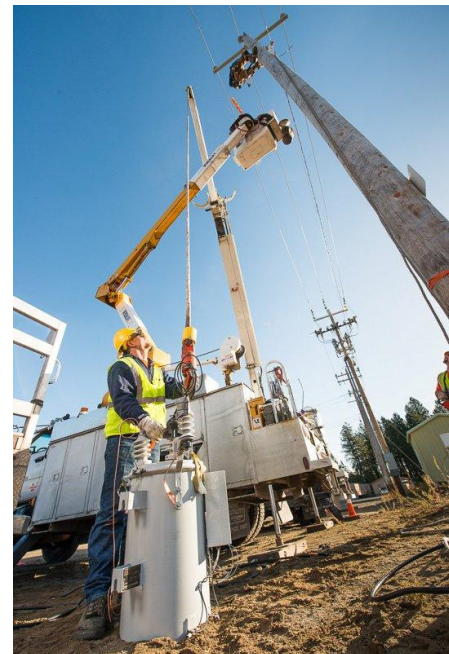
Smart transformer installation
