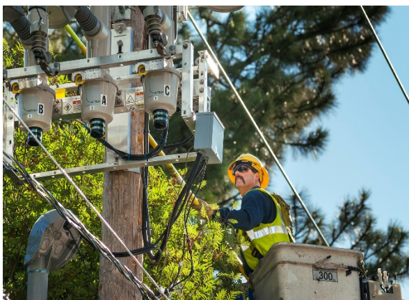
Field installation of recloser devices
