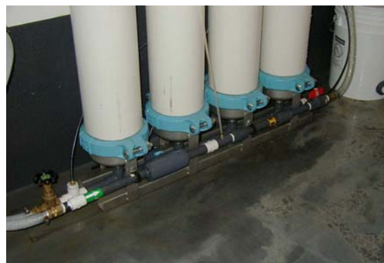
The picture on the left shows one set of filters. Source water enters through the hose inlet in the wall, passes through a flow meter, past a chlorine injection point, through an in-line static mixer, into the inlet manifold, down through the filter media. Product water is discharged through the wall. The pail holding the sodium hypochlorite solution can be seen to the right of the filter vessels and the in-line chlorine analyzer is on the wall above the NaOCl container. The sample ports and analytical equipment is forward of the chlorine analyzer. A second container of Ferric Chloride solution and feed pump is provided for pilot testing for arsenic removal.
