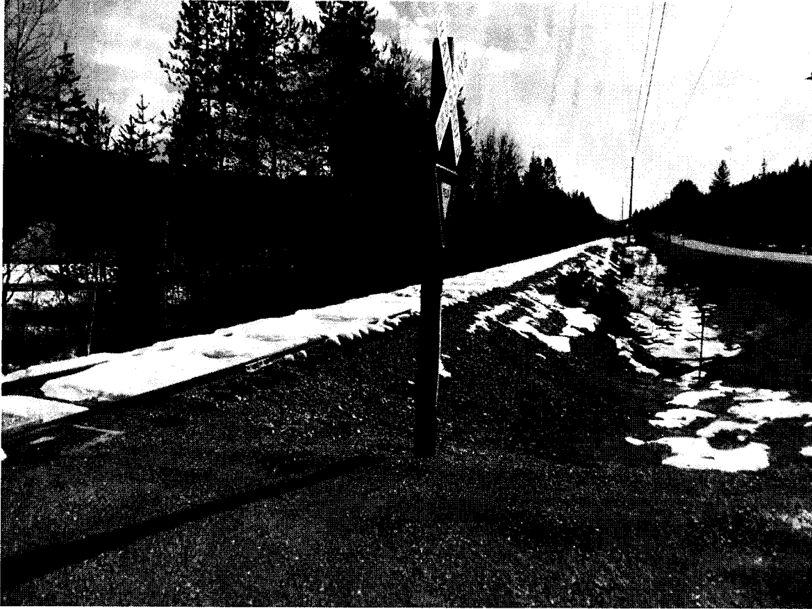
Lost Creek Drive Crossing looking South
