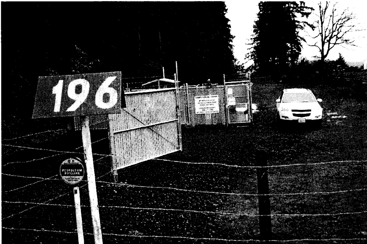
Figure 21: Mainline Valve at MP 196
