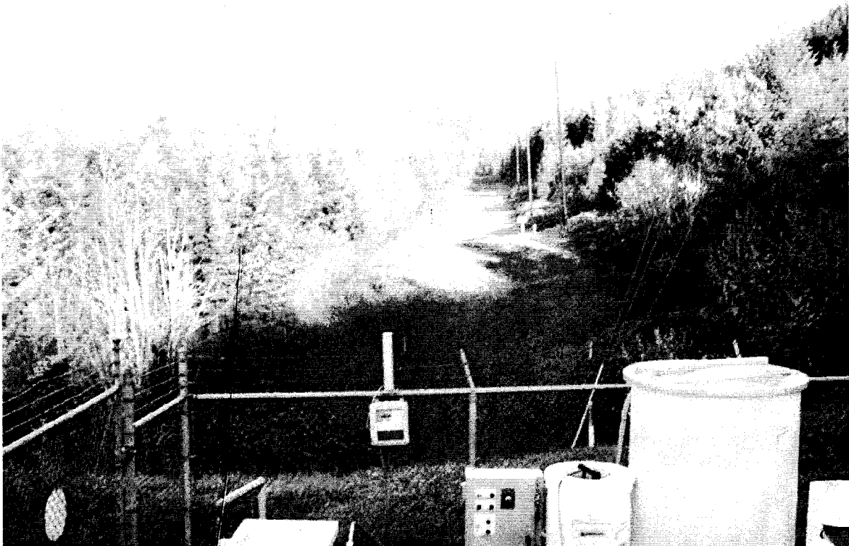
Figure 18: Pipeline right-of-way near the Castle Rock Station
