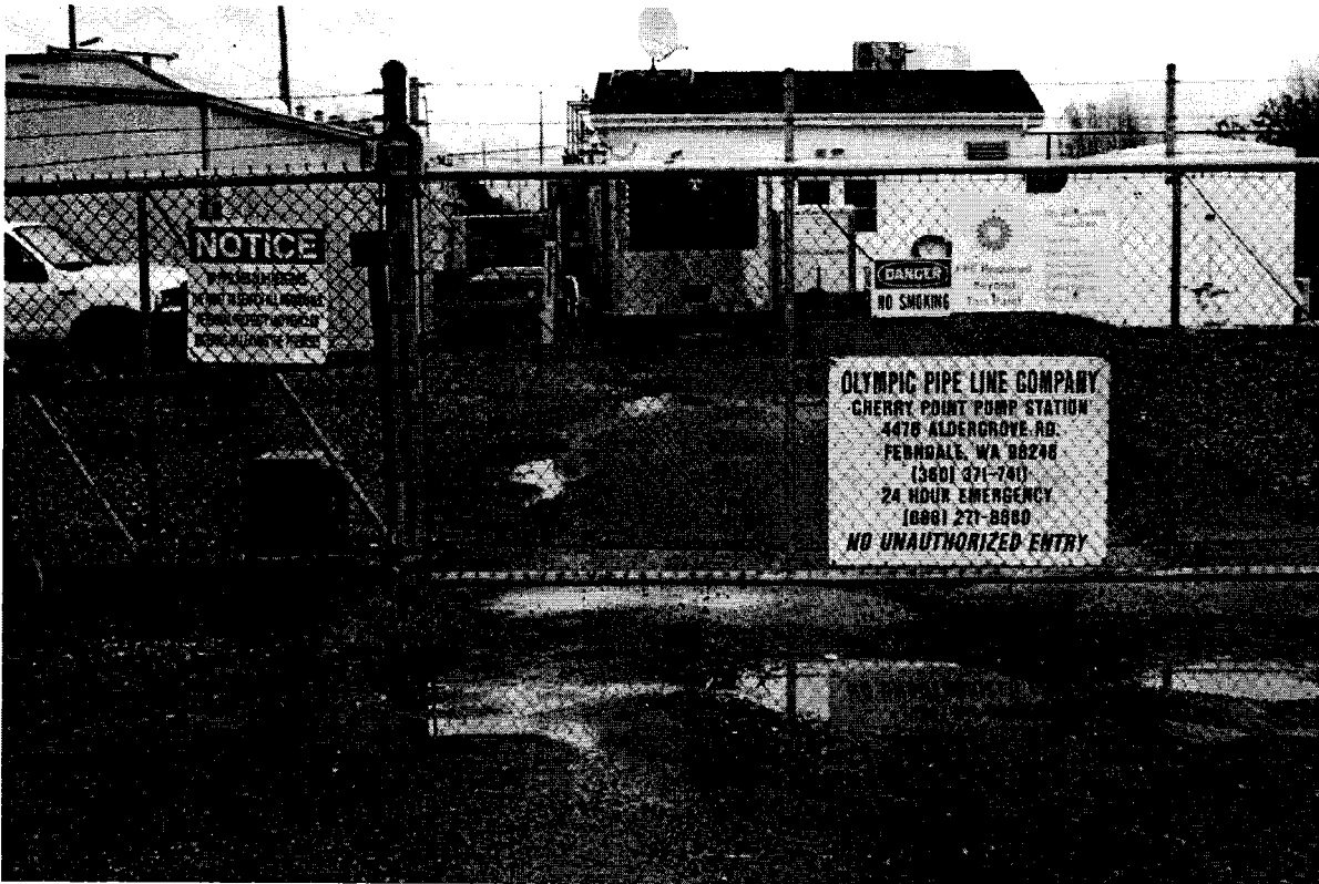
Figure 3: Signage at the Cherry Point Booster Station
