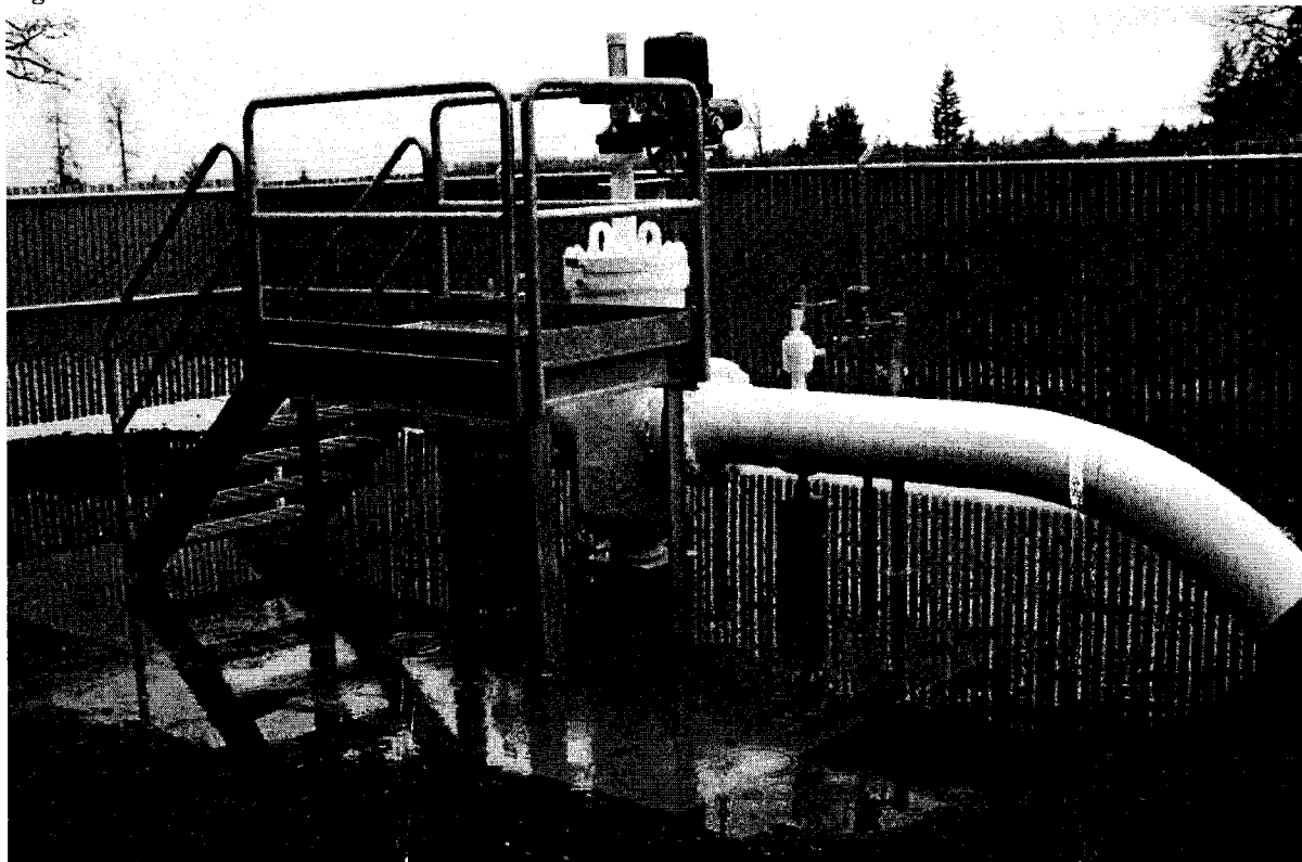
Figure 22: Mainline Valve at MP 196
