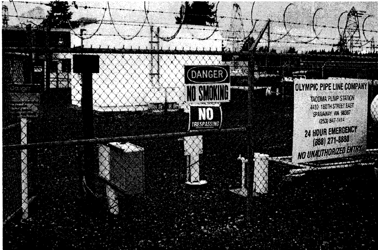
Figure 14: Signage at the Tacoma Pump Station
