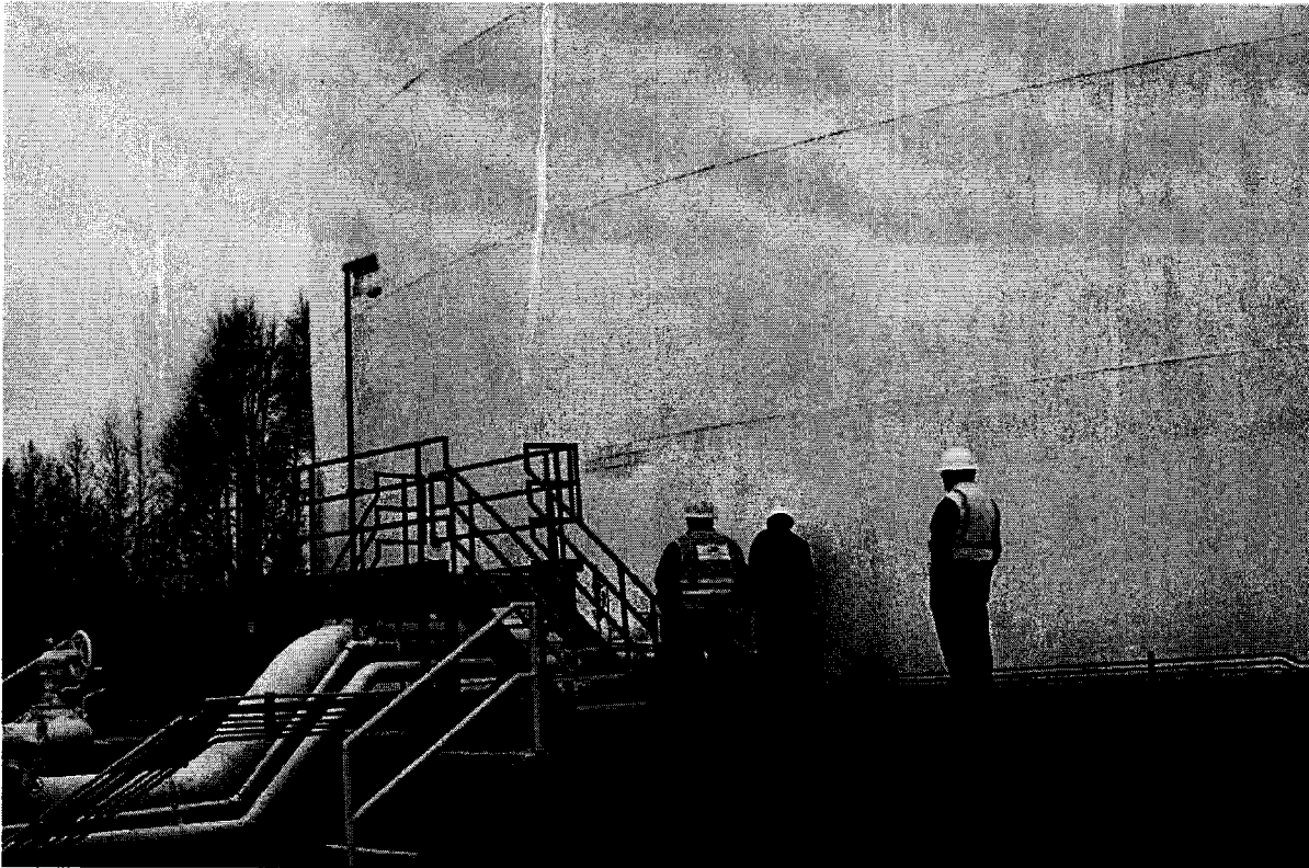
Figure 7: Breakout Tank at the Bayview Terminal
