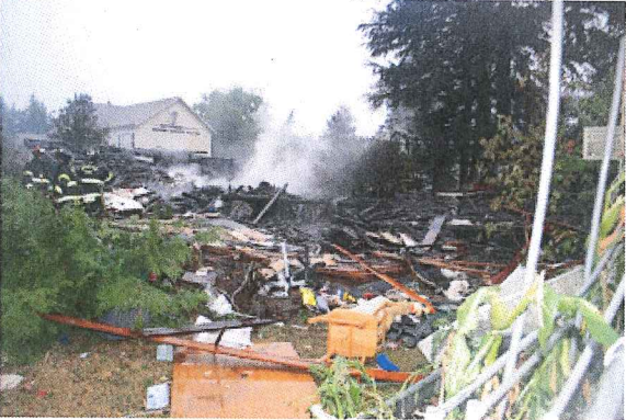
21. explosion site – from s.e.corner →n.w.
