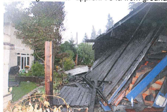
20. west side of garage – looking north
