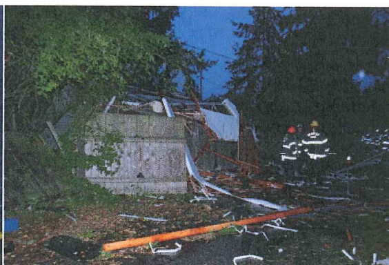
4. "alley" ->west – damage to s. neighbor fence
