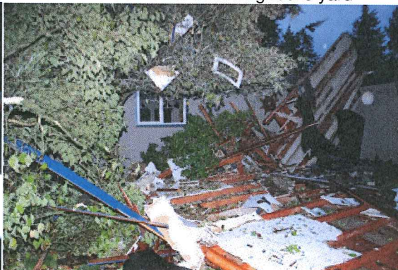
8. east neighbor – note large wall sections
