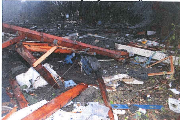
22. gas meter – s.e. corner of house →north
