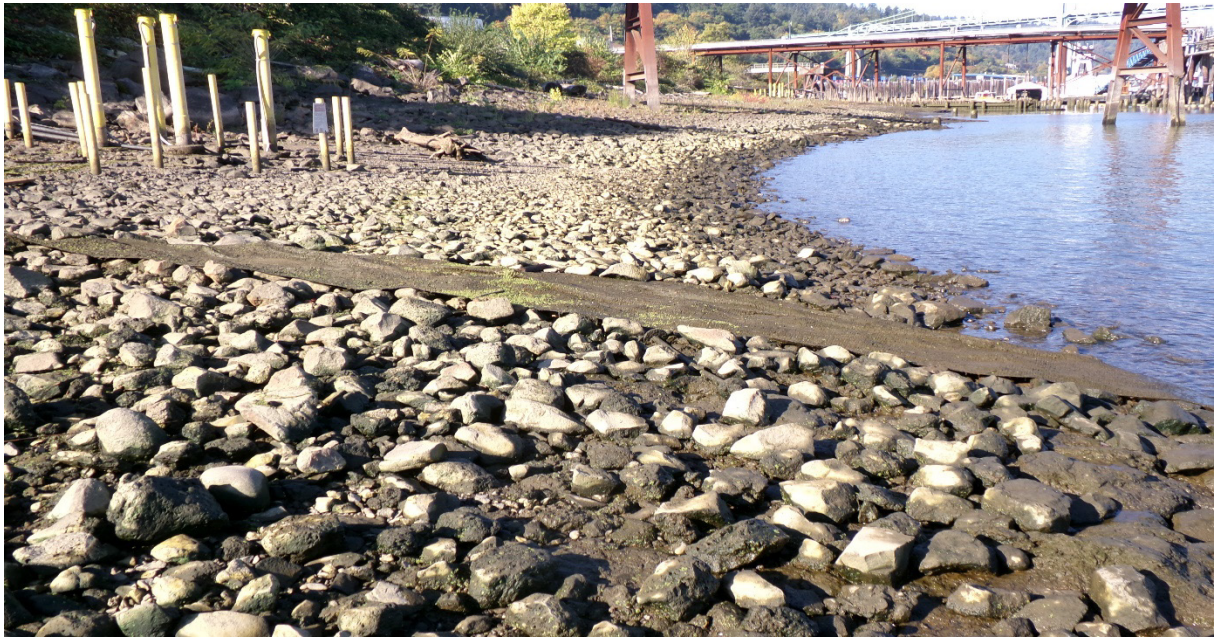
Photo 2 Organoclay Mat Material at the Upriver Extent of the Cap Area (10/27/2023)
