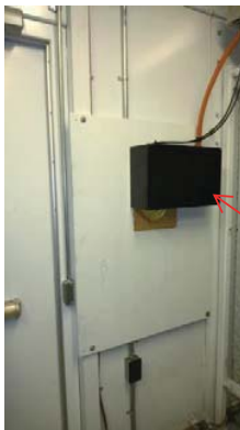
Turbine Fiber Distribution Panel - Located in substation control
