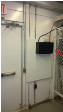
Turbine Fiber Distribution Panel - Located in substation control
